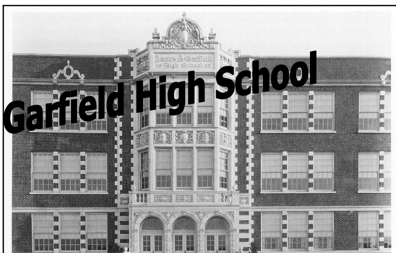
Garfield High School is one of the historic schools scheduled for modernization to be completed by 2008 under the BEX II Program
