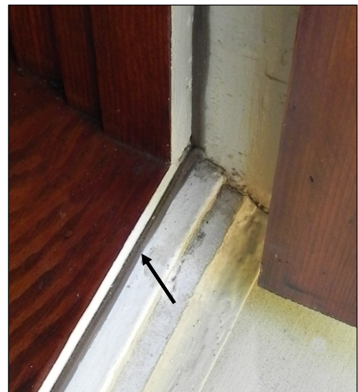
Compression weather stripping on a wood casement window.
