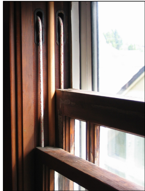
Unpainted jambs decrease friction and allow window sashes to open and close more easily.
