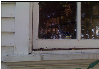
Example of a window that will not close completely because it is racked
