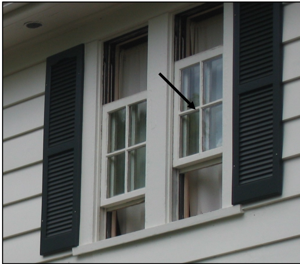
Example of muntins on a pair of historic wood windows. Photo courtesy of Patty Spencer
