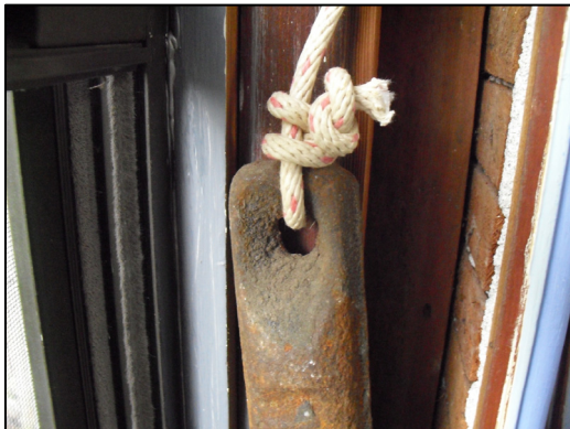
Example of a properly knotted sash cord.
