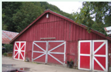
Stuart Landing Barns 103040 Carnation-Duvall Road, Carnation 1920-50
