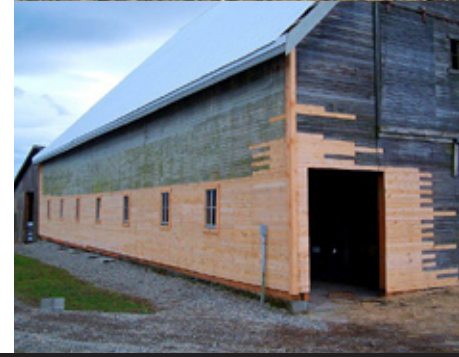
About 15 feet of the foundation of the East Barn wall is missing. The wall is dangling.
