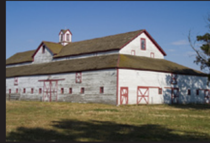
Gable-on-Hip Barn (gable roof surrounded on all four sides with a hip roof)
