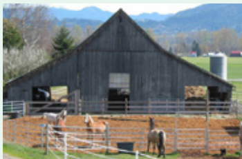
Whiting Barn 18402 Dry Slough Road, Mount Vernon circa 1900
