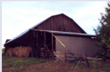
Van Eaton Farm Thomas Cobb Van Eaton Barn 11310 Eatonville Hwy, Eatonville 1914
