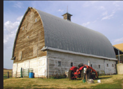
Gothic Barn (pointed arch roof truss)
