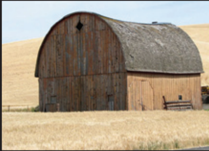
Bow Truss Barn (completely arched roof trusses)
