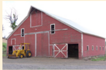
Hancock Farm 102 Carpenter Road, Prescott 1917
