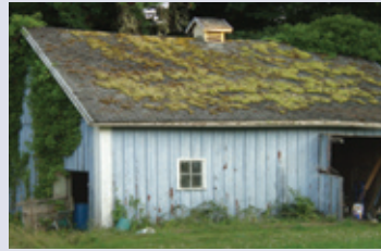
Carlson Farm August Carlson Barn 252 Island Boulevard, Fox Island 1906
