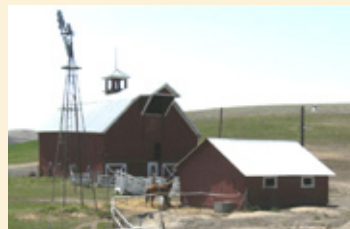
Gordon Farm James Gordon Barn 13301 Pine City Road, St. John 1906
