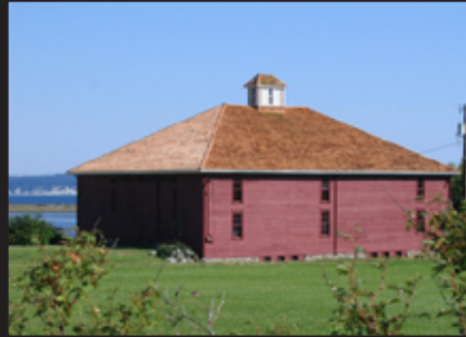
Hip Barn (sloped roof on all four sides of structure)
