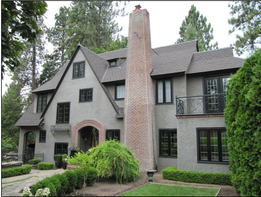
2 of 20 East façade of house in 2015 WA_Spokane County_Christensen House_0002.tif
