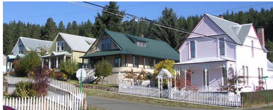
East Addition Gable Front and Cross Gable
