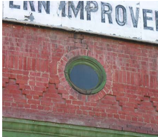
Brick detailing NWI General Store
