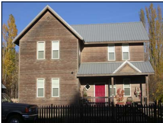
New construction, residential
