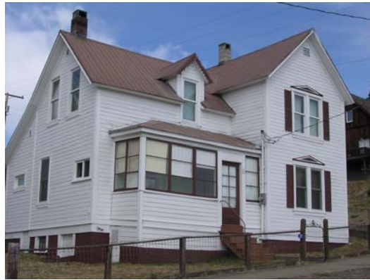
Rear shed roof addition and enclosed porch
