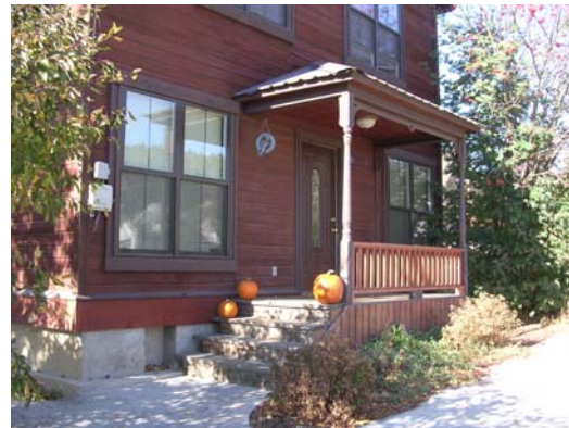
New construction, residential
