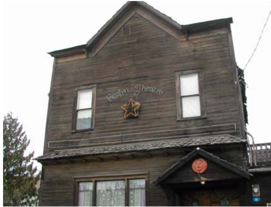
Roslyn Theatre formerly town Mortuary Western Vernacular with falsefront
