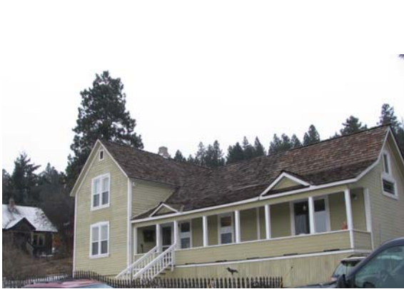
Right half of wing is new addition
