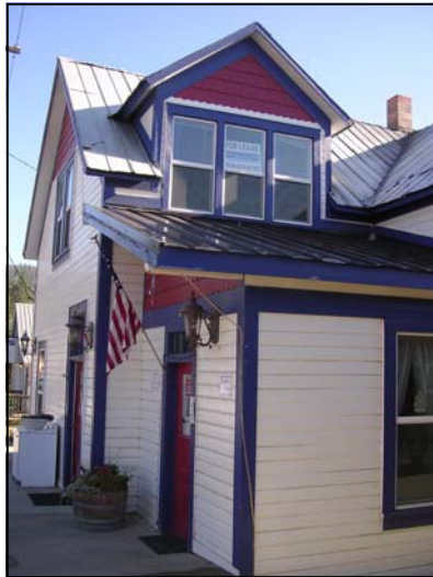
Rehabilitation, commercial Former VFW Hall
