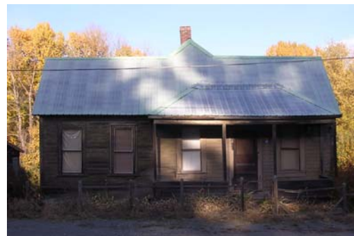
South Addition Side Gable
