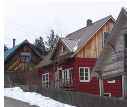
Second story addition
