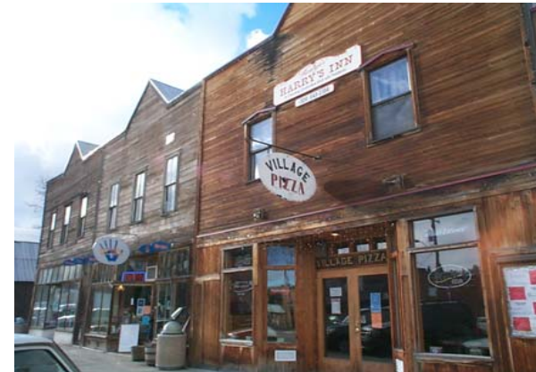
Harry's Inn is new construction.
