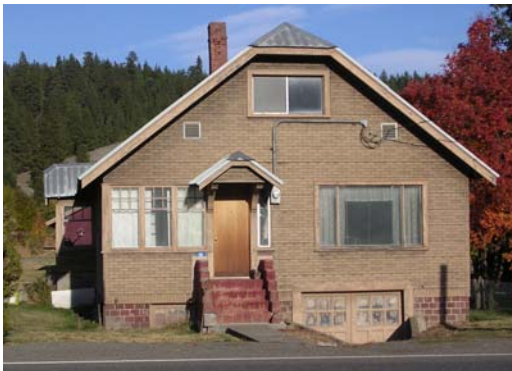
South Addition Gable Front
