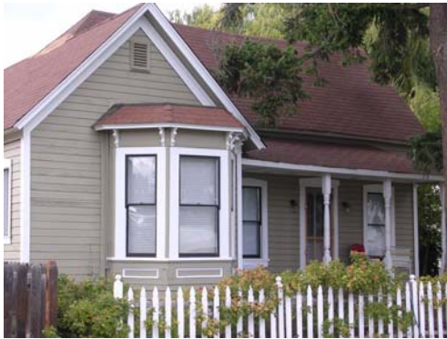
Original Town Gable Front and Wing
