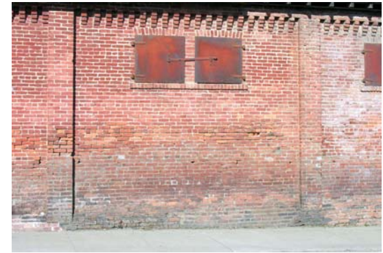
Brick detailing NWI General Store
