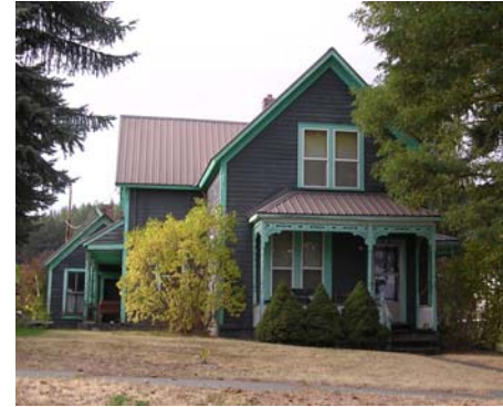
Original Town Gable Front and Wing
