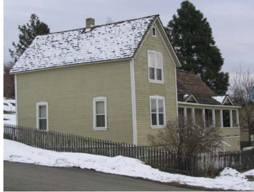
East Addition Gable and Wing Brassington House
