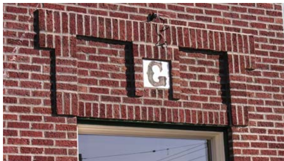
Brick detailing Masonic Hall
