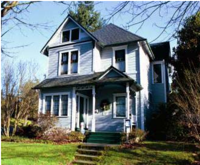
Example of historic window and door trim at 329 Avenue B.
