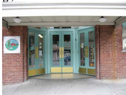
Appropriate lighting under a built awning at the building entry of 902 First Street.
