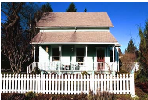
Shed roof at entry porch on parapet a cross gabled house
