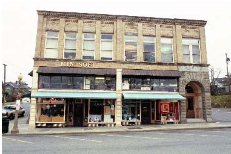
An example of first floor ceiling heights that are taller than upper story heights at 1024 First Street.
