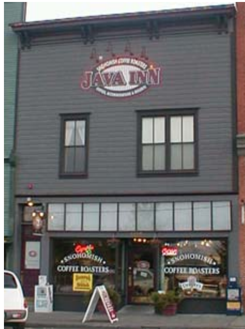
An example of approved signage with lighting at 1120 First Street. See detail on page 36.
