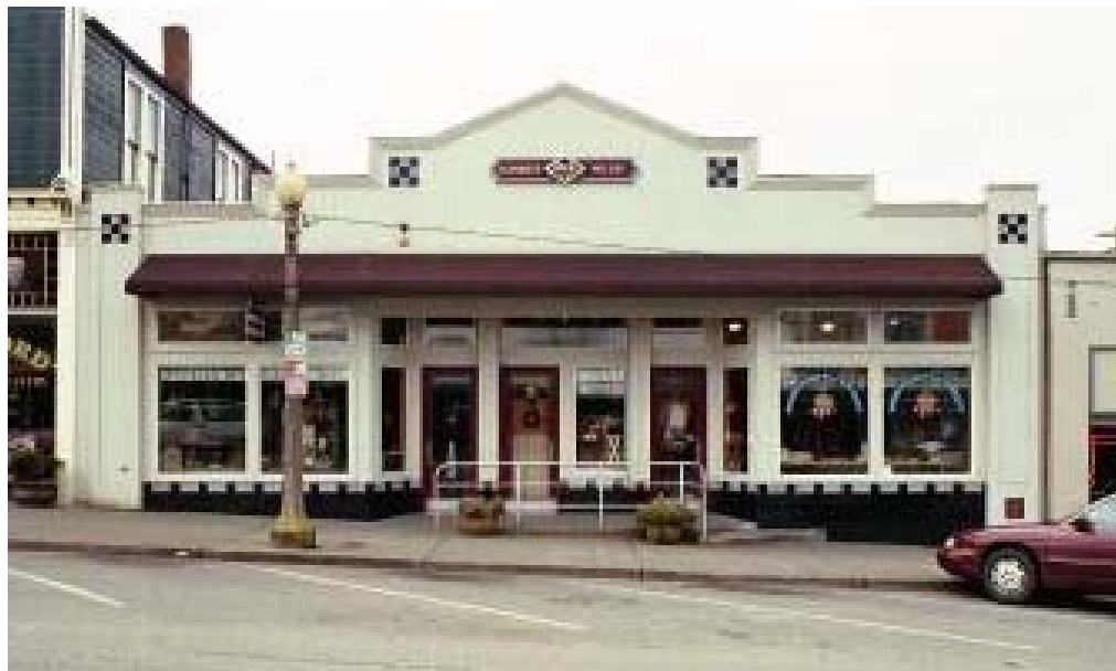
An example of new construction at 915 First Street that is consistent in style and is appropriately modulated and scaled relative to other historic structures on First Street.
