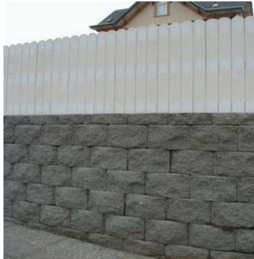
An example of acceptable masonry block with decorative surface.
