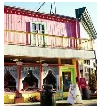
Flat roof – note cornice at the right
