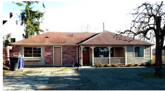
205 Avenue C Cross Hipped roof on a Ranch style house
