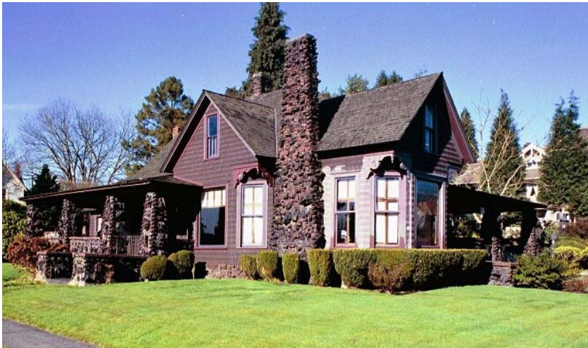
An example of traditional building materials: wood and brick. The irregular “clinker” brick is shown in this example at 304 Avenue D.
