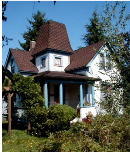
232 Avenue G Mansard Roof at tower over entry - The main part of the house is cross Gabled.
