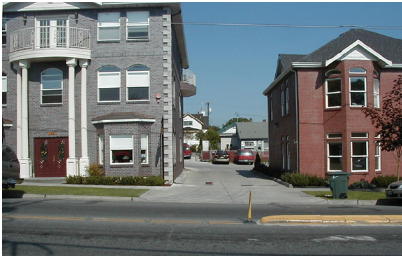
An example of new commercial construction with shared driveways and parking behind. 209 Avenue D is on the left and 207 Avenue D is on the right.
