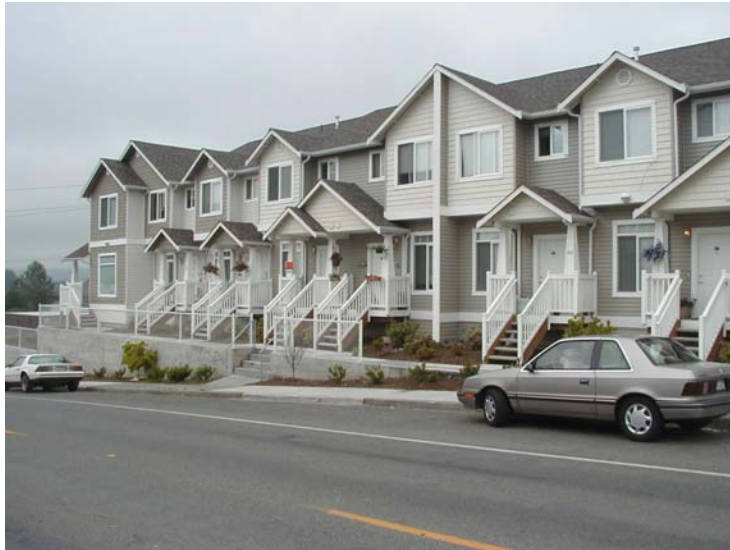
An example of sidewalks provided to each entry of a multifamily project without crossing a parking lot located at 105 Lincoln.
