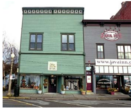
1122 First Street Flat roofs with parapets
