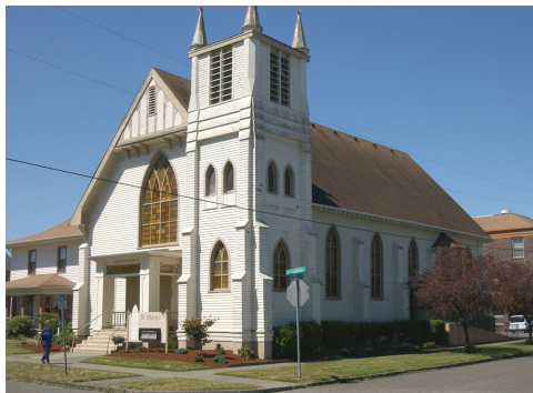
St. Mary's Church, Centralia - 1910
