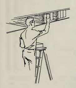
Plywood sheets (2' x 8' x ½" cut to fit) should be securely fastened to the joists using 2 inch, #8 screws 10 inches apart. Bricks or blocks are then packed as tightly as possible into the openings between the joists. Be sure to fill as much space as possible. To get the most protection out of this improvement, one-quarter of the basement ceiling over the best corner should be filled with bricks or solid concrete blocks.
