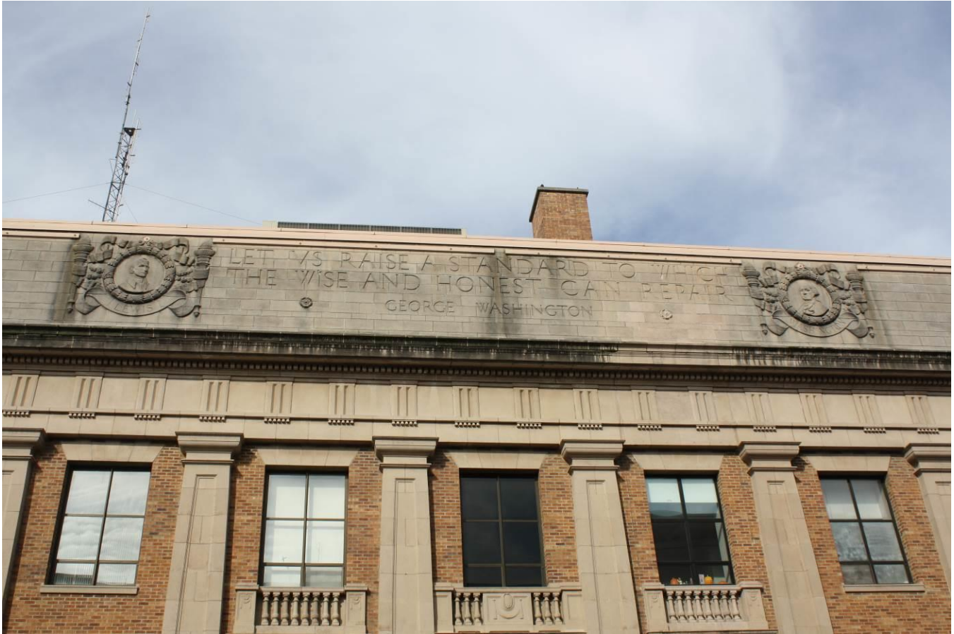
LewisCounty_HistoricCourthouse_007 Cornice Detail – north facade
