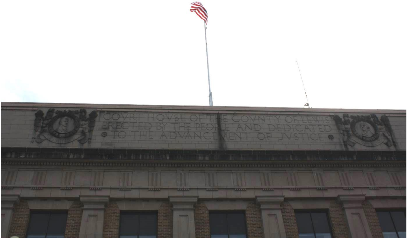
LewisCounty_HistoricCourthouse_006 Cornice Detail – south facade
