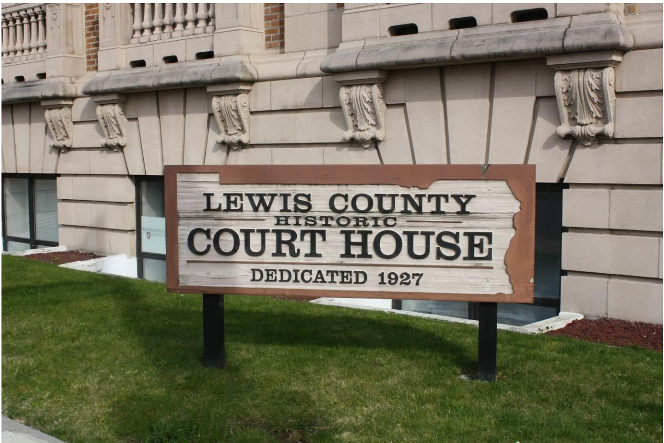
LewisCounty_HistoricCourthouse_005 Window sill detail
