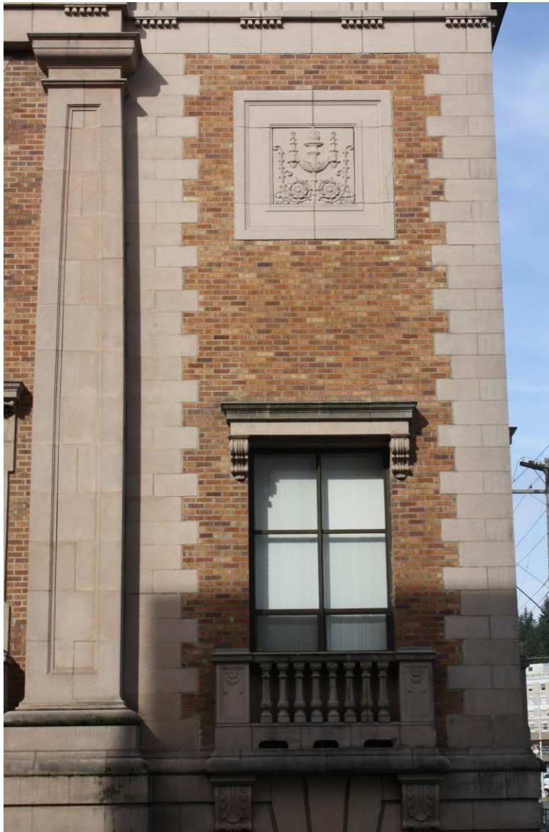
LewisCounty_HistoricCourthouse_009 Facade Detail – SE corner
