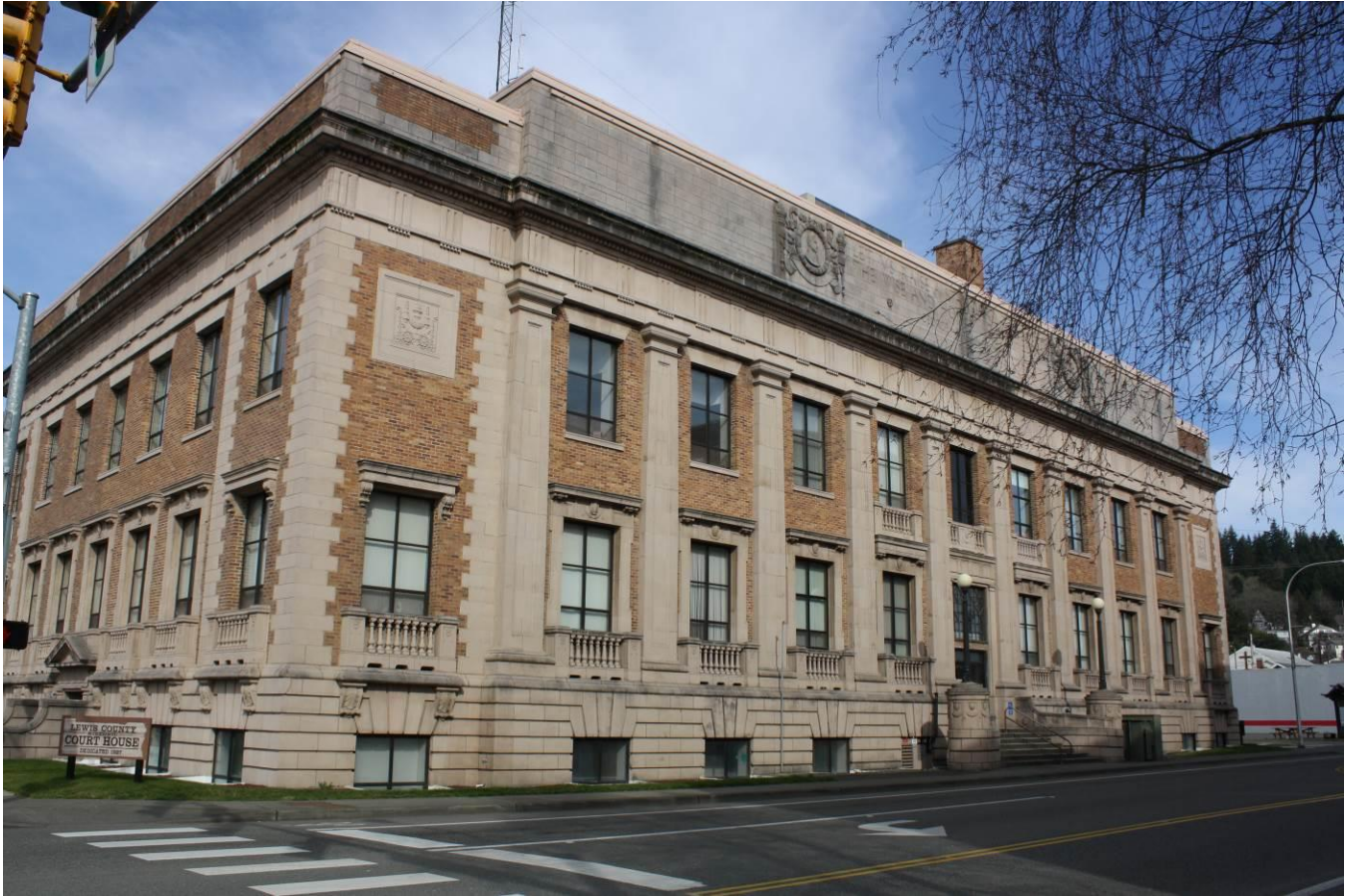
LewisCounty_HistoricCourthouse_004 South (Main Entry) Facade
