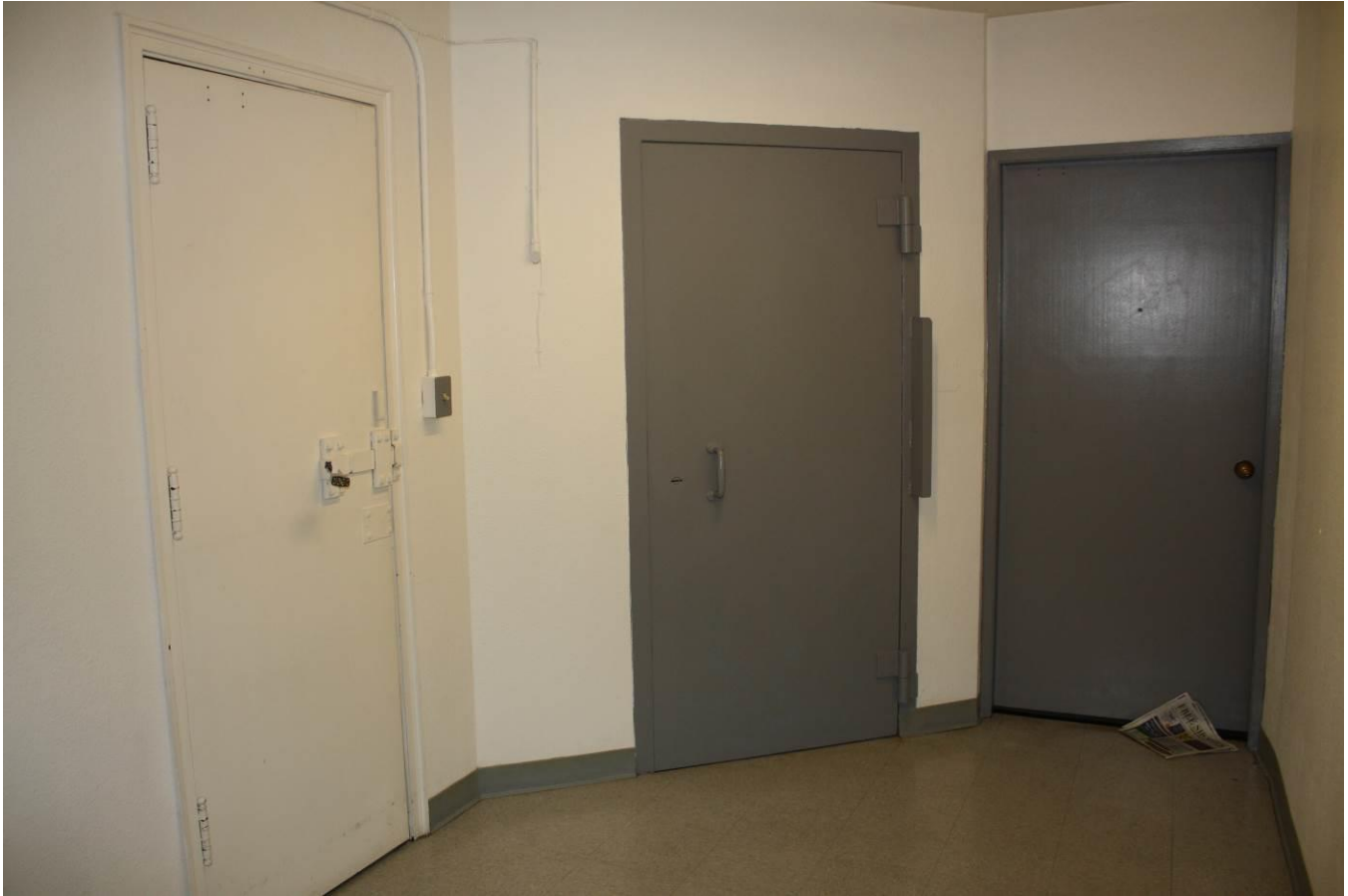
LewisCounty_HistoricCourthouse_020 Third Floor jail doors
