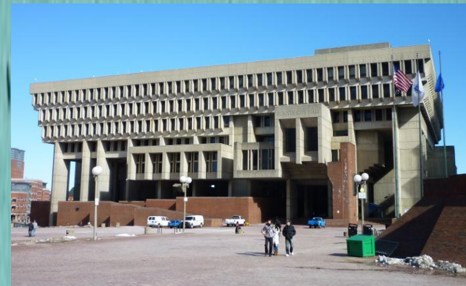
Boston City Hall Kallmann, McKinnell and Knowles, Boston, 1963-68
