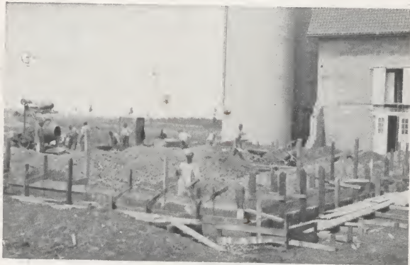
Building the foundation.
