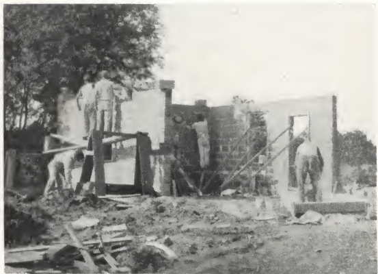
Completing the walls of a fireproof, permanent two-car garage.
