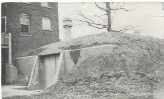
Concrete combines rotproofness, water tightness, and great strength and is therefore universally used for storage cellar construction.
