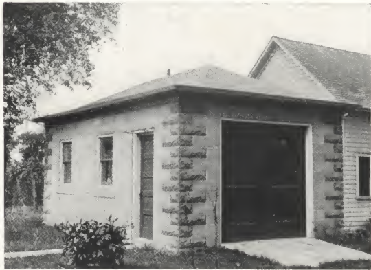
Maximum fire protection is afforded by the garage built of concrete.
