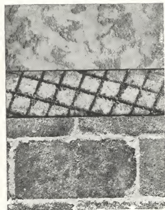
Portland cement stucco applied to concrete masonry wall—construction that both permanent and attractive.
