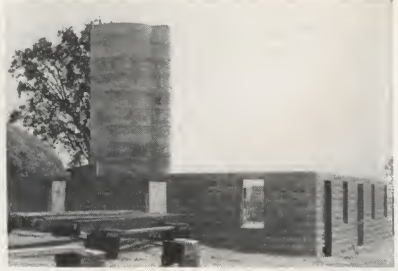
Concrete masonry units lay easily and quickly and take only a small amount of mortar.
