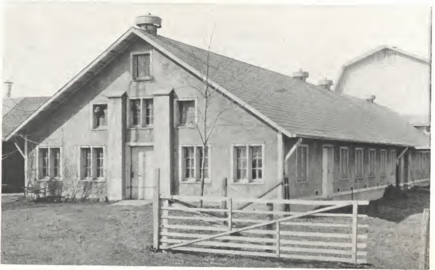
An abundance of sunlight, uniform temperature, a plentiful supply of fresh air, and the highest possible degree of cleanliness, make this one-story, concrete barn ideal for housing dairy cattle.
