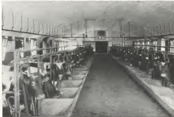
The utmost degree of sanitation is made possible when the dairy barn floors and mangers are made of concrete.
