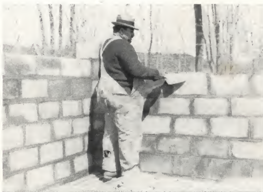
Concrete masonry units make speedy erection possible.
