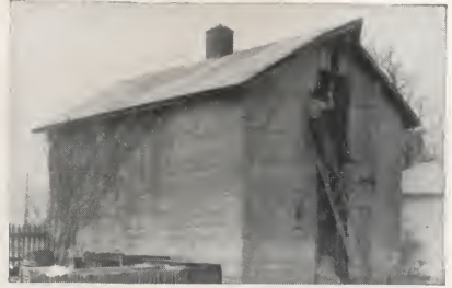
Because of its fireproof and rotproof qualities, concrete is well adapted to icehouse construction.
