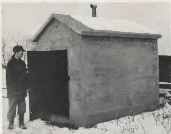
Smokehouse fire dangers are eliminated by concrete construction.
