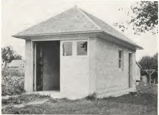
Concrete garages withstand severe wind storms.
