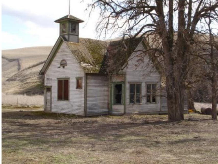
Northwest façade in 2008 at original site
