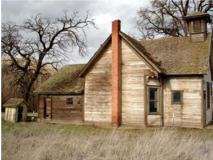
East facade in 2008 at original site
