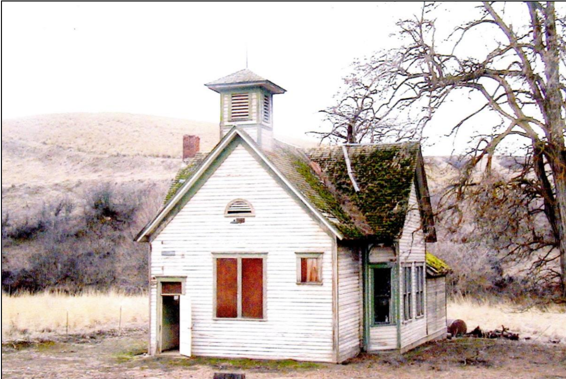
North façade of Smith Hollow School in 2008 at original site
