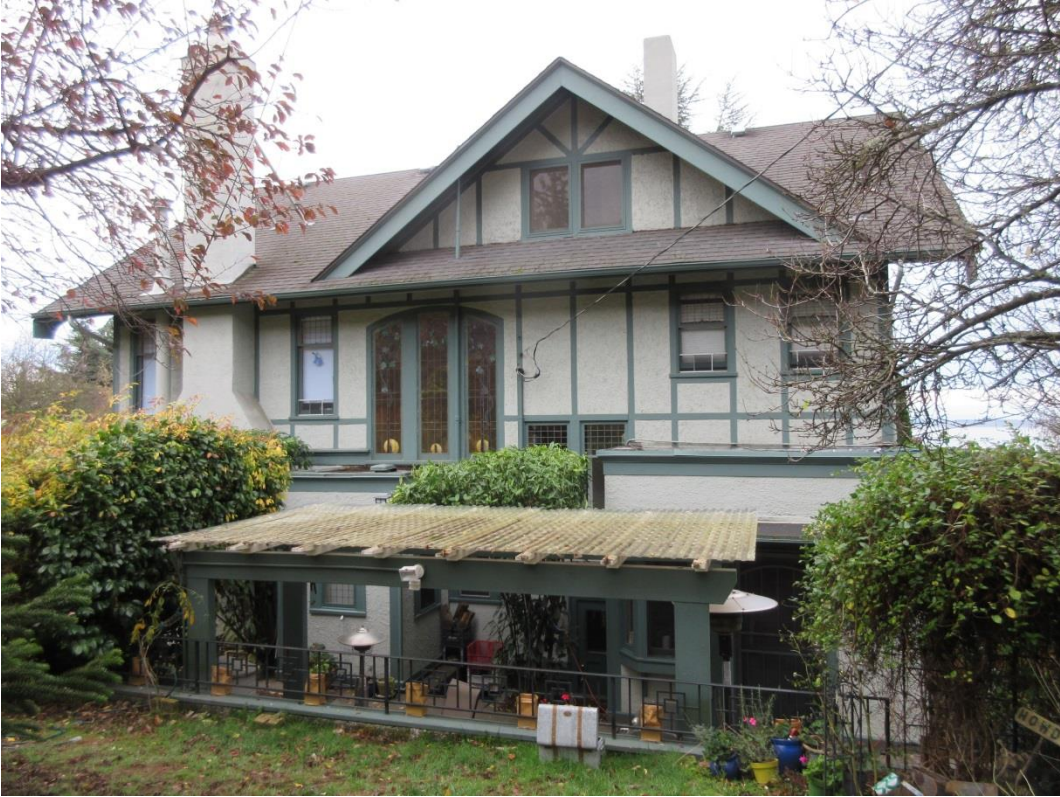
4 of 11 East Elevation showing rear of house with art glass window on second story
