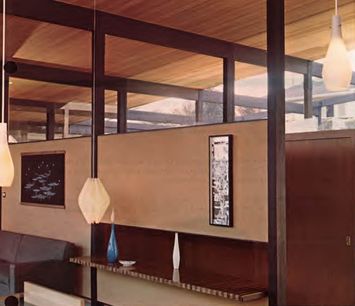
Materials used in modern post and beam structures must be selected with care. They must be structurally sound and look good too. Here Western Red Cedar roof decking is left exposed for warmth and beauty. Grade: "B & Btr." Pattern: Double Tongue and Groove, "V" Joint. Grain: Vertical Grain. Finish: Semi-transparent stain.
