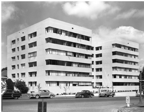
28 – Capitol Center Apartments 1517 Capitol Way S Architect: Fred Rogers, 1949
