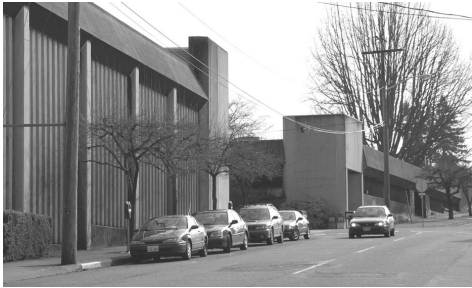
19 – State Parking Garages Union Ave & Columbia St Architect: Warren Brown, 1958 & c.1972
