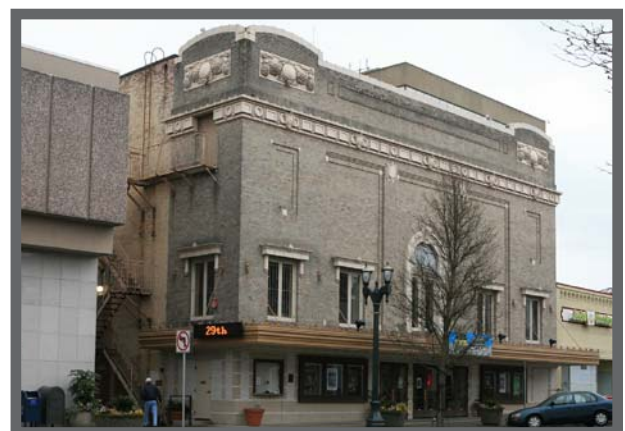
Masonry structure (Everett Theatre, Everett). Source: Artifacts Consulting, Inc. 2008.
