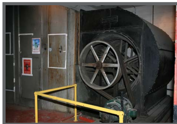
Historic operational ventilation system. Source: Artifacts Consulting, Inc. 2008.
