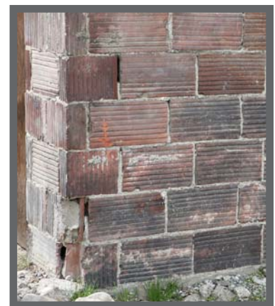
Detail of a hollow clay tile exterior clad wall. Source: Artifacts Consulting, Inc. 2008.
