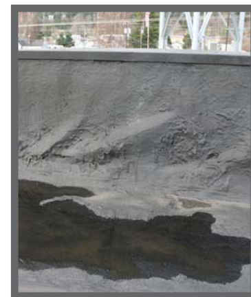
Roofing with holes and pools. Source: Artifacts Consulting, Inc. 2008.
