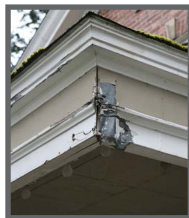
Damaged metal entrance canopy. Source: Artifacts Consulting, Inc. 2008.
