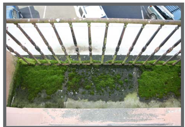
Looking down at an exterior balcony covered in moss. Source: Artifacts Consulting, Inc. 2008.
