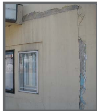
Stucco needing repair. Source: Artifacts Consulting, Inc. 2008.
