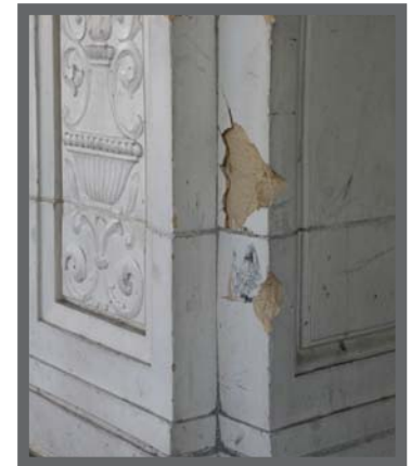
Detail of damaged terra cotta. Source: Artifacts Consulting, Inc. 2008.
