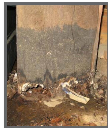
Deteriorated wood post. Source: Artifacts Consulting, Inc. 2008.
