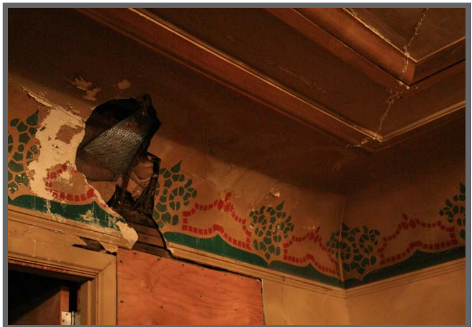
Interior plaster walls and ceilings often show localized water damage, usually from a past roof leak. Source: Artifacts Consulting, Inc. 2008.
