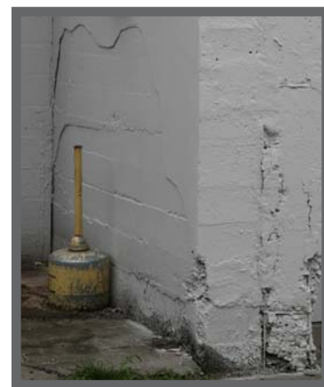
Example of shallow rebar, too large aggregate in early concrete work. Source: Artifacts Consulting, Inc. 2008.
