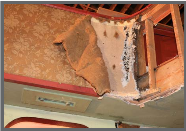
Detail of silk covered sound baffling which has deteriorated from moisture and coal dust saturation over many years. Source: Artifacts Consulting, Inc. 2008.
