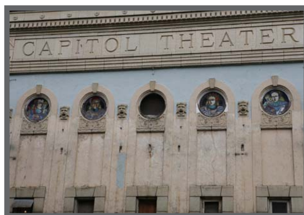
Facade detail showing missing stained glass window, damaged stucco. Source: Artifacts Consulting, Inc. 2008.
