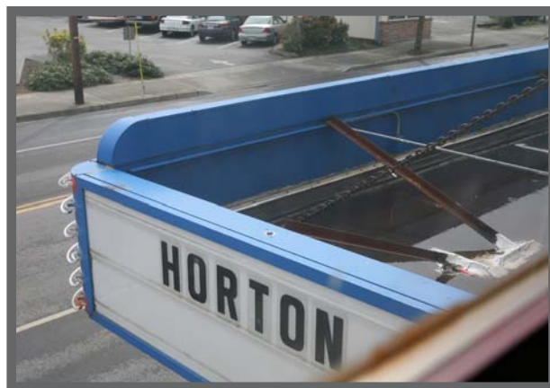
Detail of a canopy marquee with standing water. Source: Artifacts Consulting, Inc. 2008.
