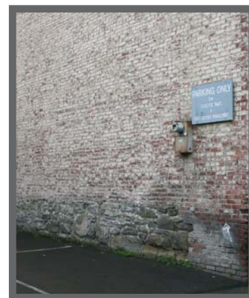
Stone and brick foundation. Source: Artifacts Consulting, Inc. 2008.
