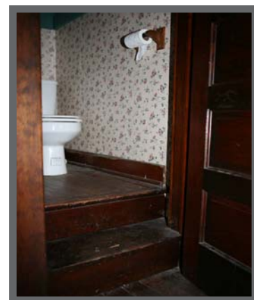
Non-ADA compliant restroom. Source: Artifacts Consulting, Inc. 2008.
