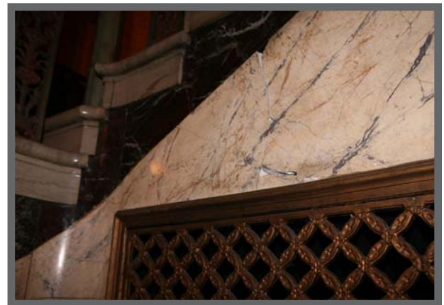
Detail of broken stone veneer lining a stairwell. Source: Artifacts Consulting, Inc. 2008.
