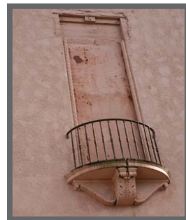
Restoration of various facade elements needed (missing shed roof, rusting metal rail, boarded over windows). Source: Artifacts Consulting, Inc. 2008.
