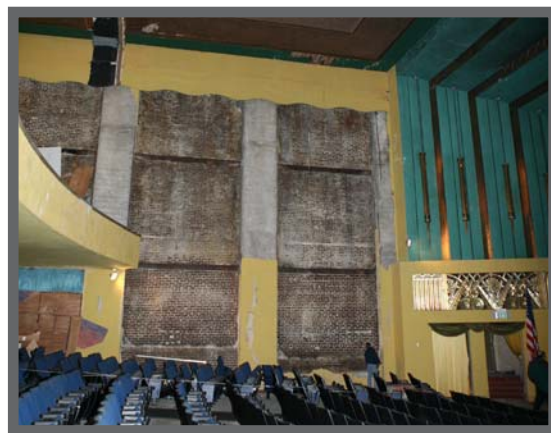
Composite concrete and brick structure (Fox Theater, Centralia). Source: Artifacts Consulting, Inc. 2008.
