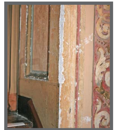
Damaged proscenium arch plaster. Source: Artifacts Consulting, Inc. 2008.
