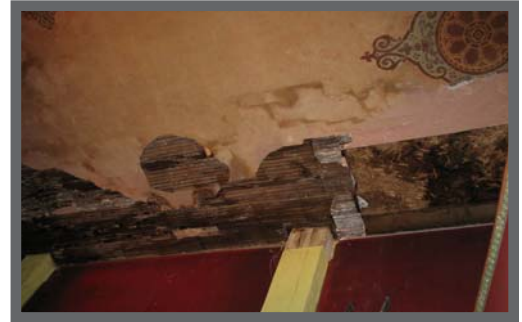
Stabilization of interior plaster ceiling needed. Source: Artifacts Consulting, Inc. 2008.
