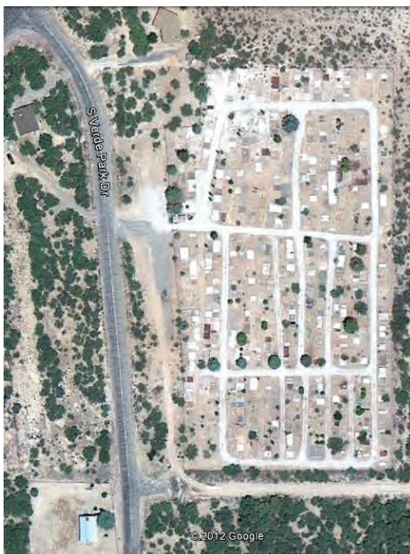
Figure 4: Clear Creek Cemetery and Church (at lower left) at Camp Verde, Arizona Image from Google Earth
