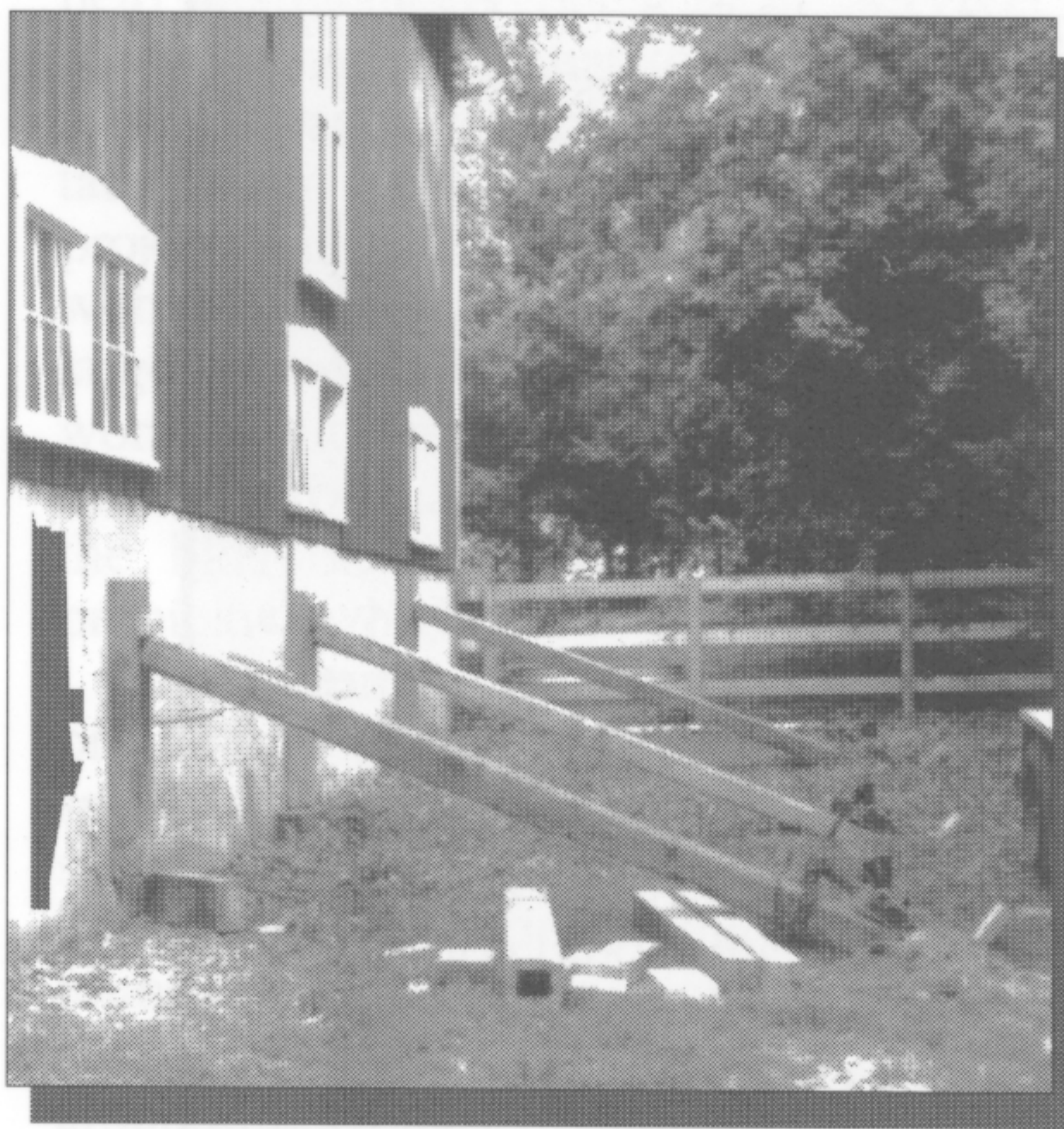
Jacks used to push a concrete wall back into place.
