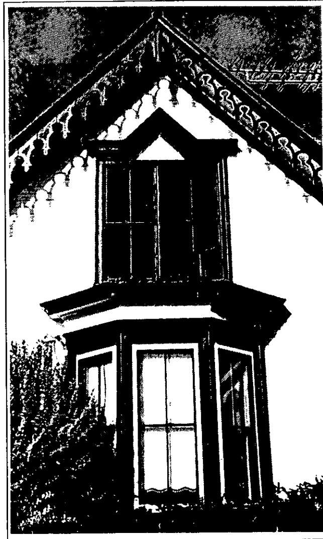
Gable roofs are dominant forms in most Oysterville buildings. (Tom Crellin House)
