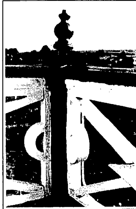
Ornament and detail of historic buildings add visual interest to the community. (Tom Crellin House)
