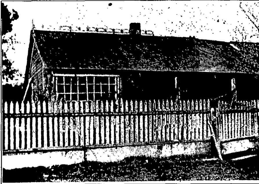
Decorative trim along the ridge of the Wert House once added an ornamental accent. Reconstruction of such elements is appropriate when such photographic evidence exists.
