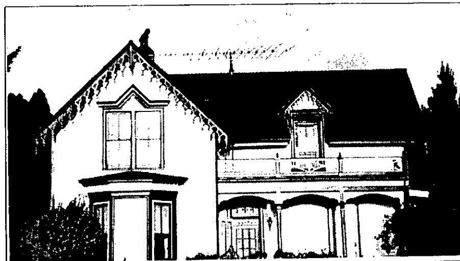
Preserve original roof forms. (Tom Crellin House, 1869)
