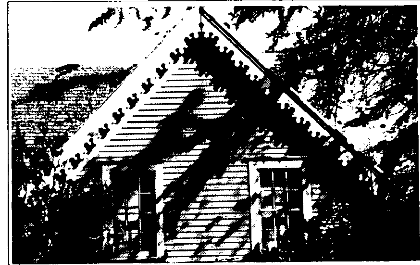
Decorative barge boards in the gable ends of the John Crellin House, late 1860's, give it a distinct identity, even though its basic form and materials are similar to others in the district.
