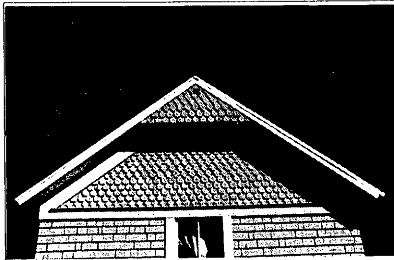
Generally, decorative shingles are appropriate only in gables and on dormers. (D. C. Stoner House)
