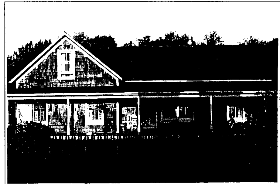
Roofs shall be similar in form to those of historic residences. (W.D. Taylor House, early 1870's)
