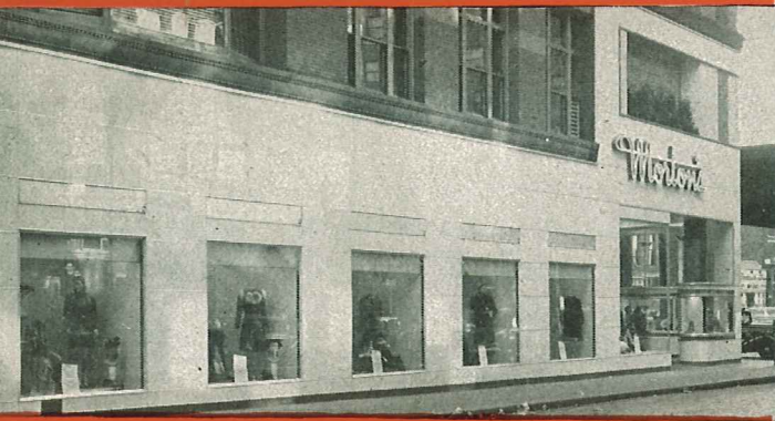
Typical store modernization in an old building
