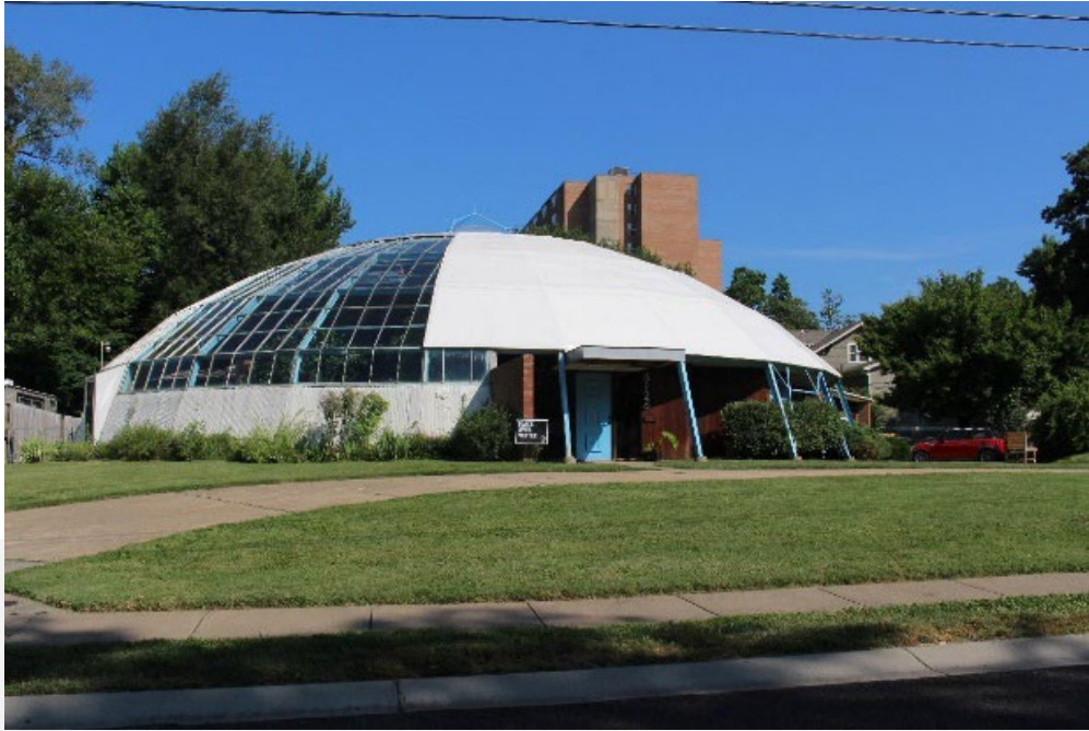
100009040 Campbell Dome House, Montgomery County, Kansas. This photograph is an example of exterior image showing primary facade, setting, materials, and design.
