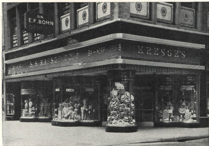
S. S. Kresge Co., Cleveland, Ohio Trim on front windows, trim on front, flashing and canopy over sign of Enduro. Background of sign is Porcelain Enamel
