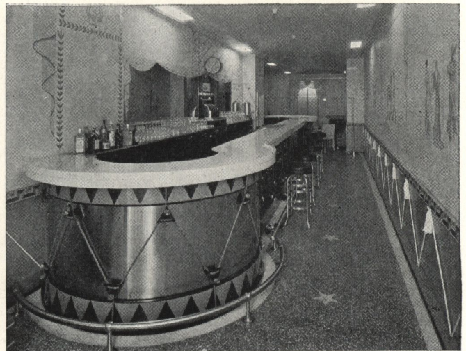
McDoel's, Inc., Buffalo, N. Y. Designer—M. J. Bernhard Co. Enduro for back of bar, panels on front, wall panels and all bright metal
