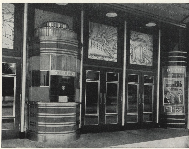
Bromley Theatre, Philadelphia, Pa. Architects—Thalheimer & Weitz Ornamental plaques, poster frames and drinking fountain of Enduro. Ticket booth of Porcelain Enameled Iron with Enduro strips
