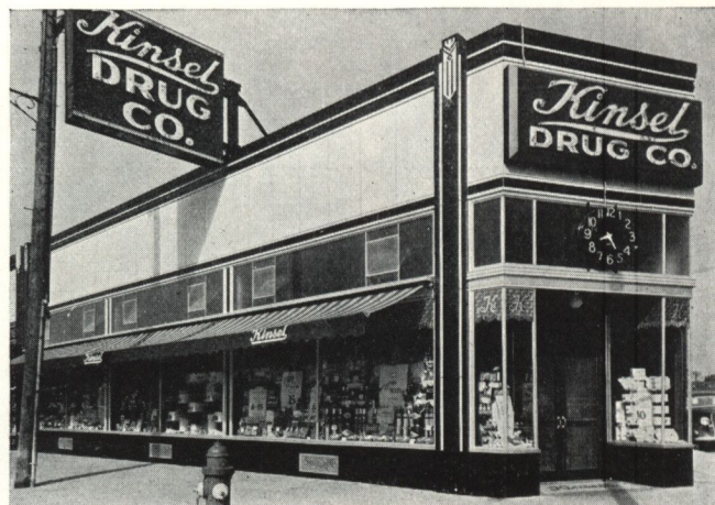
Kinsel Drug Store, Detroit, Mich. Architects—Pollmar, Ropes & Lundy Enduro used for edging on Glasiron Macotta
