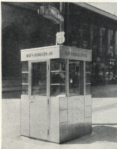
Public Information Booth, Canton, Ohio. Enduro for exterior walls, doors, sash and etched acknowledgment plate
