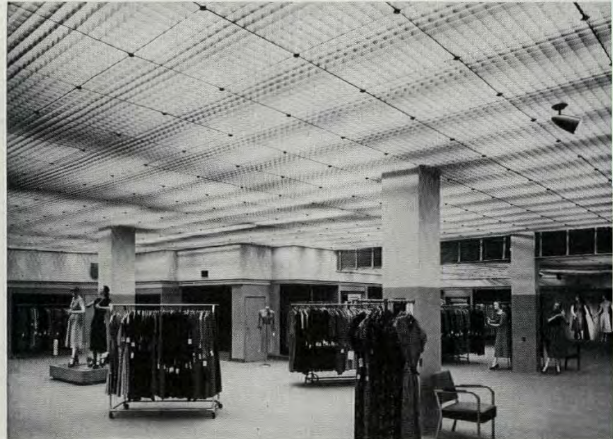
FLUORESCENT LAMPS above ceiling deliver 75 foot-candles to the sales space below. Shadowing could have been reduced by setting lamps at 45 ft. angle to louvers. All pictures: Herpolsheimer's.
