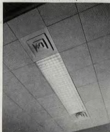
UN ADMINISTRATION BUILDING uses dry-built ceiling which incorporates air diffuser designed to ceiling module. Manufacturer has recently redesigned square diffuser to get a throw approximating 360° thus eliminating previous objections to square diffuser's tendency to streak ceiling.
