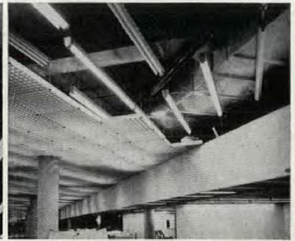
LOUVERS are engaged by star-shaped leveling device and hung from 48 in. rods.
