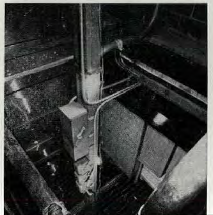
FLUORESCENT LAMPS above ceiling deliver 75 foot-candles to the sales space below. Shadowing could have been reduced by setting lamps at 45 ft. angle to louvers. All pictures: Herpolsheimer's.
