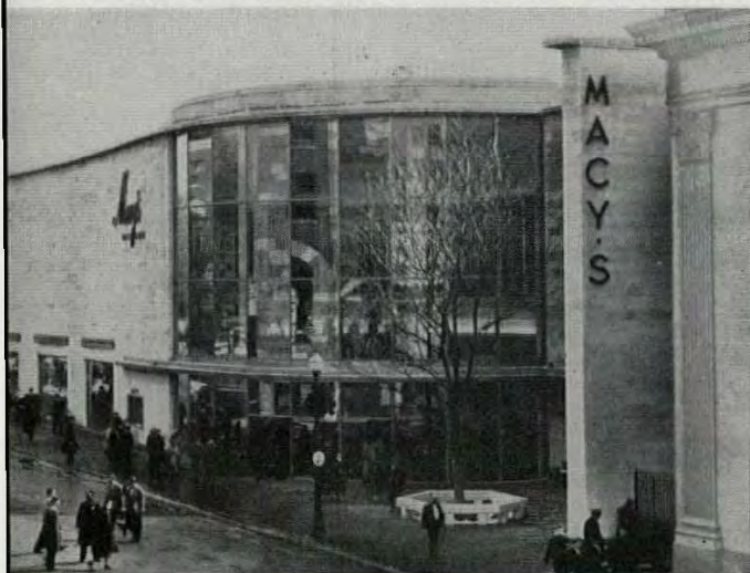
TWO-STORY OPEN FRONT in suburban store above is completely veiled by reflections. Inside second floor this much day-lighting creates obscuring glare. Macy's, White Plains.
