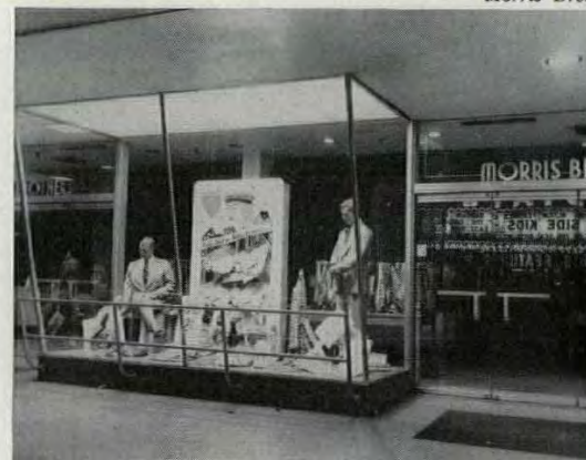
GLASS CAN BE SLANTED to reflect lower brightness surface (street shaded by overhang), giving display better visibility. Diagram (L.) shows how high-intensity lighting is used inside store to counteract daylight glare. Morris Bros., Miami Beach. Kenneth Welch.
