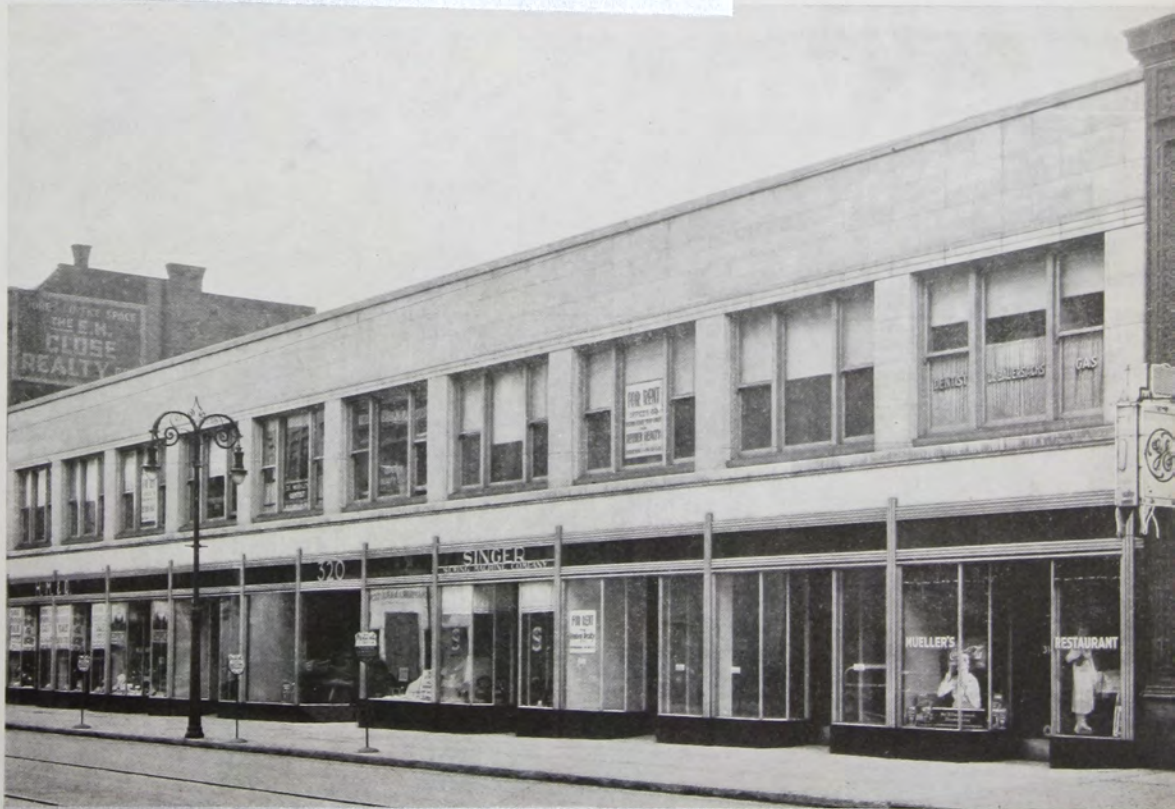
A beautiful transformation with simplicity and dignity the forethought. White metal frames of stock patterns, including recessed awning box with a field of shining black structural glass.
