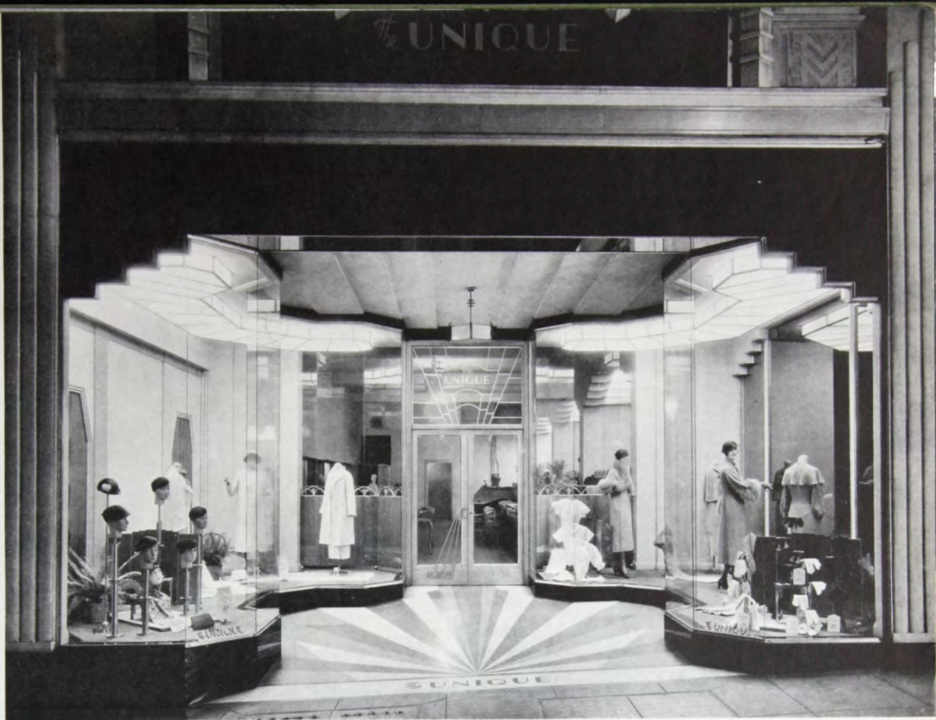
Befitting its name, only metal doors and frames present this appearance.
