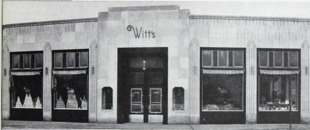
The small show windows in piers help reduce distance from main show windows to entrance.
