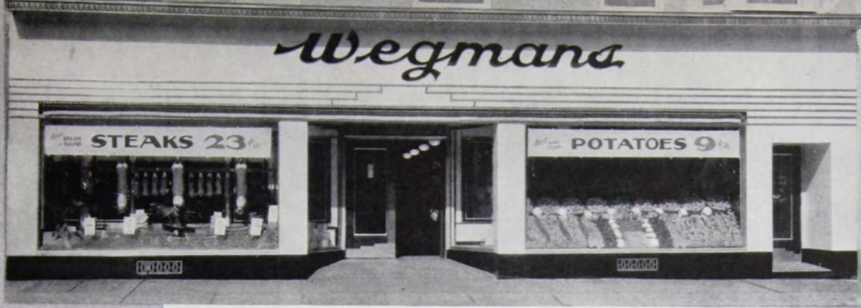
Structural columns beautifully hidden. Monotony of broad plain surface broken by metal strips.
