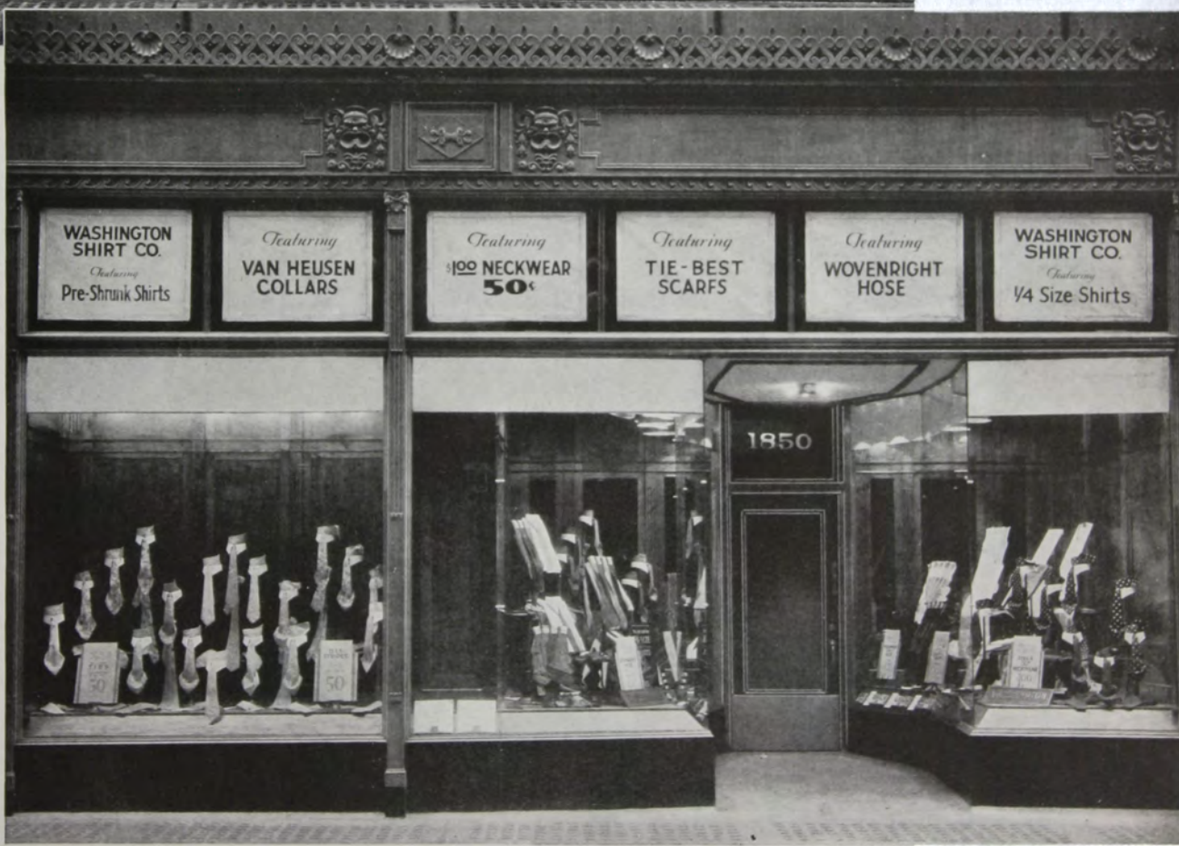
It is not always necessary to make a complete change in the front to improve its customer attractiveness. The removal of the step alone brings the entrance door nearer the shopper.
