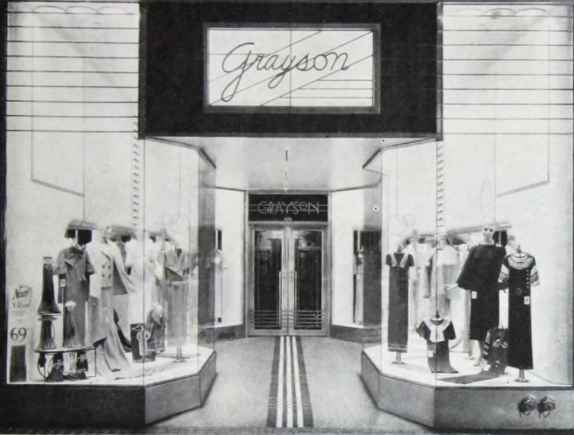
Decorative bars across upper portion of front plates add stability as well as beauty.
