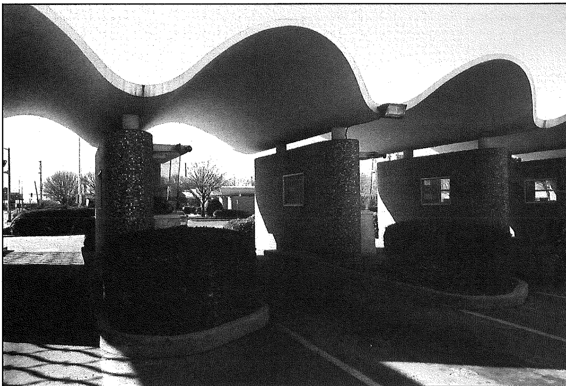
Figure 5. The concept of the drive-in as a state-of-the-art facility often inspired the use of futuristic motifs and innovative geometries. The sine-wave roof of the Central State Motor Bank (circa 1960, Wright and Selby) in Oklahoma City, Oklahoma, undulates over individual aqua-blue-mosaic-tile and brushed-metal teller booths. These were adjacent to the bank, but a matching strip of booths, perpendicular to these, was also built across the street. (The second set of booths is just visible in the background. Photograph courtesy of Ann V. Swallow.)
