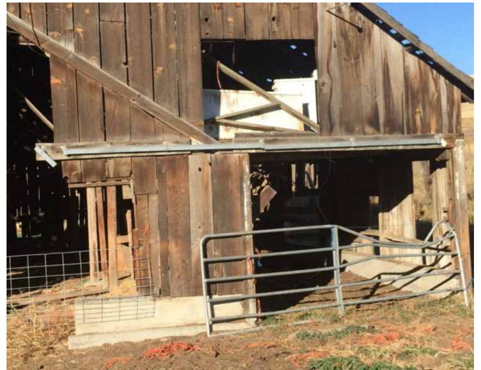
Constructed c. 1910, the structure includes a hybrid combination of round logs, hewn timbers and dimensional lumber.
