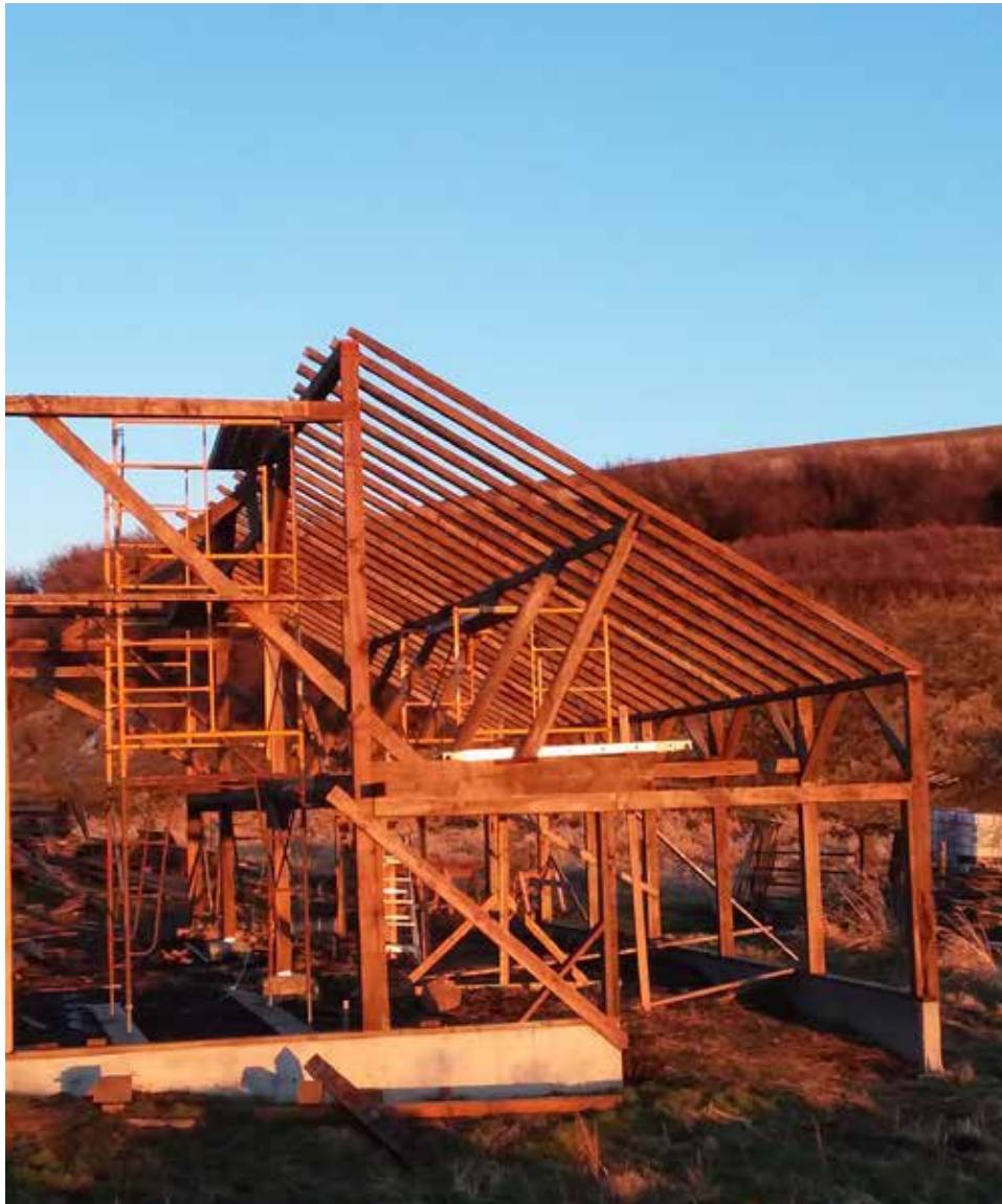
Constructed c. 1910, the structure includes a hybrid combination of round logs, hewn timbers and dimensional lumber.
