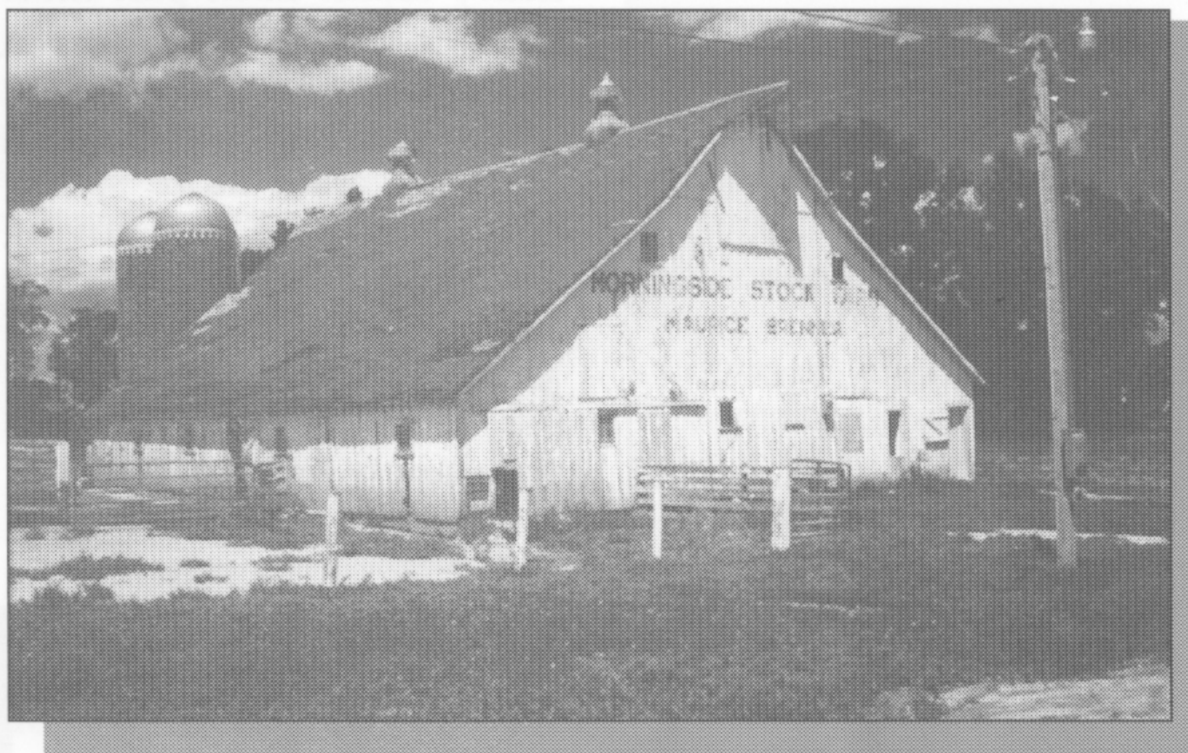
Ron Seuntjens' livestock barn, before rehabilitation for machinery storage
