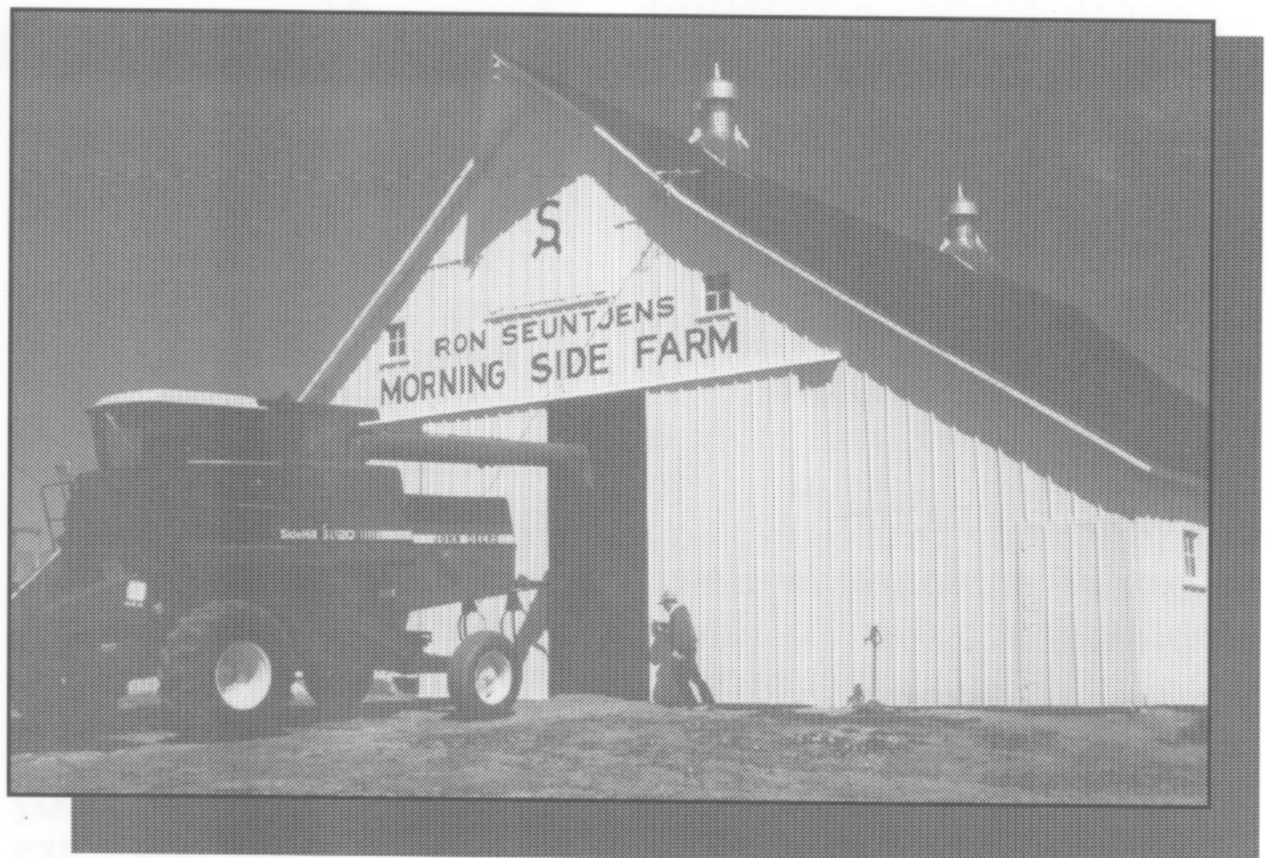
Ron Seuntjens' barn, after rehab, with sliding wood doors
