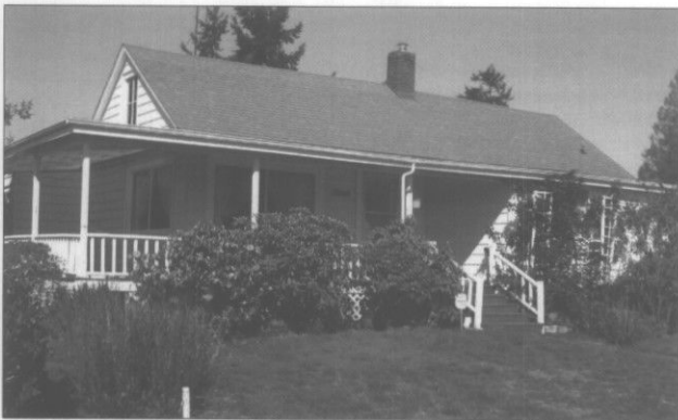
Front or wrap around porches with shed roof forms were common on beach cottages.
