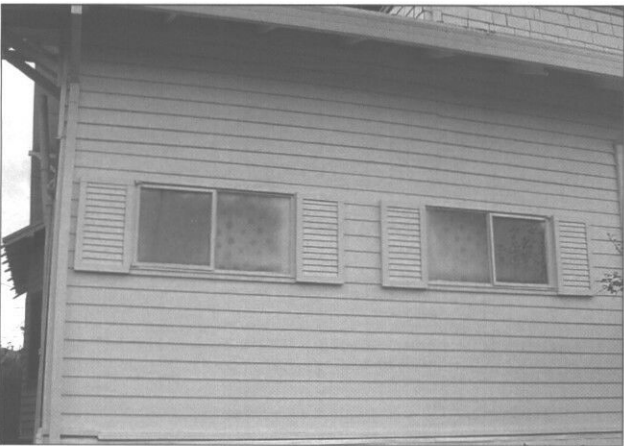
Do not add new window or door openings on character-defining facades. (Sacramento, CA)
