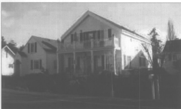
Most residential roof forms are pitched, such as gabled (pictured), hipped and gambrel roofs. (Steilacoom, WA)
