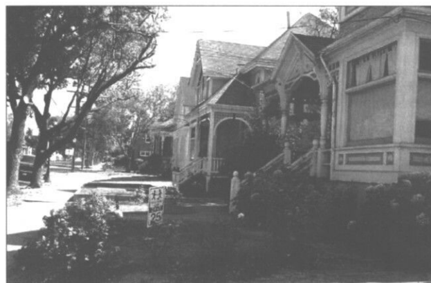
Maintain an attractively landscaped yard where residential characteristics existed historically. (Napa, CA)
