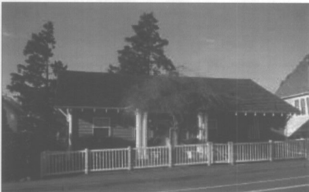
This Craftsman style bungalow at 1511 Lafayette (c. 1920) exhibits exposed rafters, knee brackets, a full width porch and clapboard siding.
