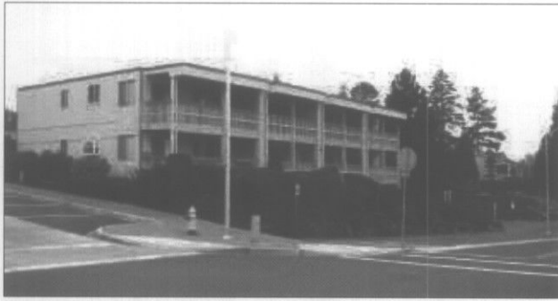
Orient a new building parallel to its lot lines, similar to that of traditional building orientations.
