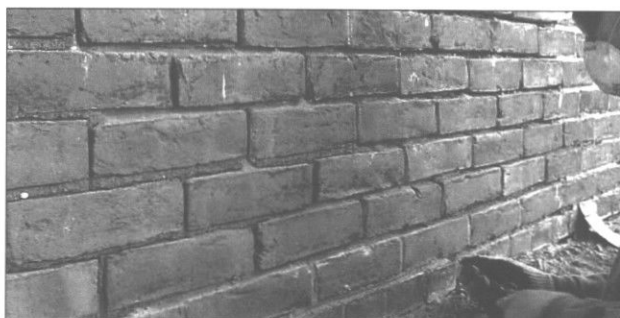
Commence with building cleaning after any repointing has completely cured.
