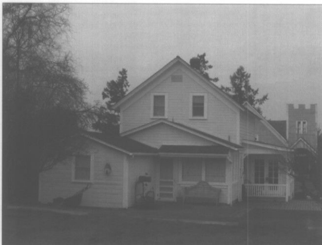
The rear additions to the Gardiner House exhibit compatible gable and shed roof forms.
