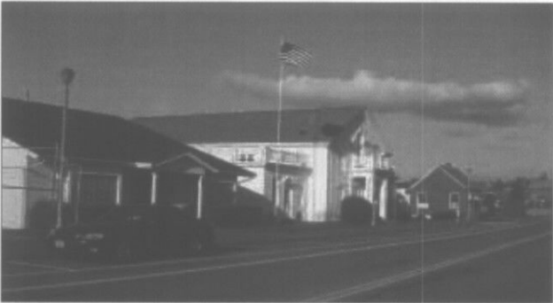
When new street lights are to be installed, they should be designed to be subtle and unobtrusive.
