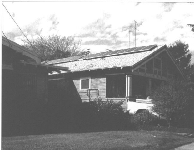
If attached to the building, solar devices should lay flush with the roof line, as seen in the photo above. The devices in the top two photos are inappropriate. (top photo: Bellingham, WA; bottom photo: Spartanburg, SC)
