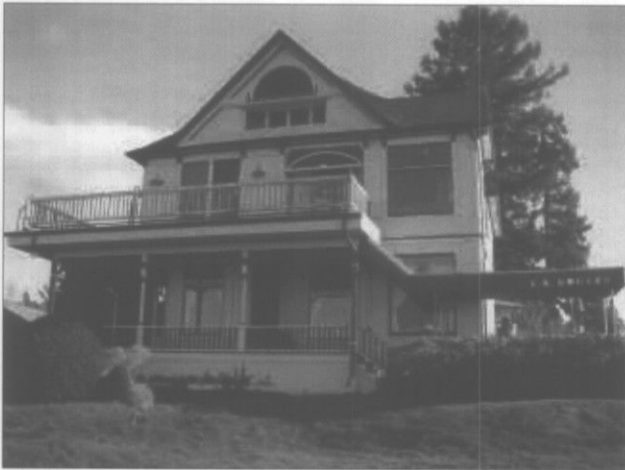
Lap siding is a typical material.
