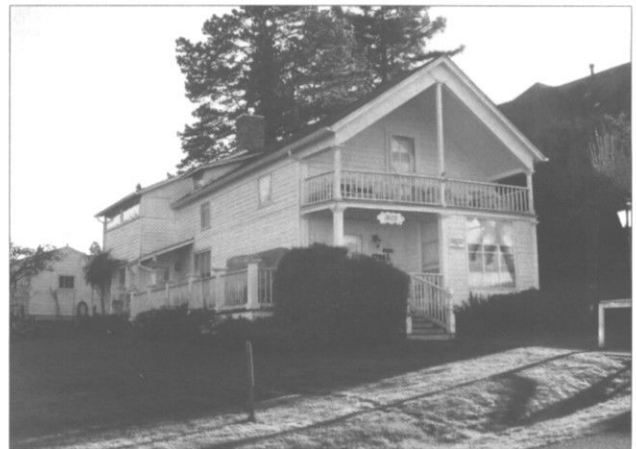
Many structures, such as the Webster House c. 1855 at 1706 Commercial Street, have experienced additions over time. This structure had an early addition that was removed in the mid-1900s (see photo at left) and retains rear additions.
