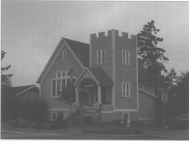
The former Oberlin Congregational Church was built in 1903 and exhibits many elements of the Gothic Revival style, such as the square tower with crenellated parapet and clapboard siding.
