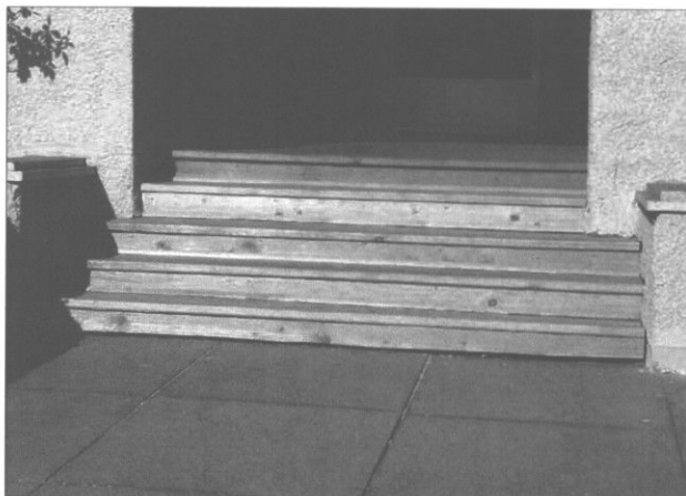
Appropriate: Use materials similar to those seen historically. Wood decking was most common. (Pasadena, CA)
