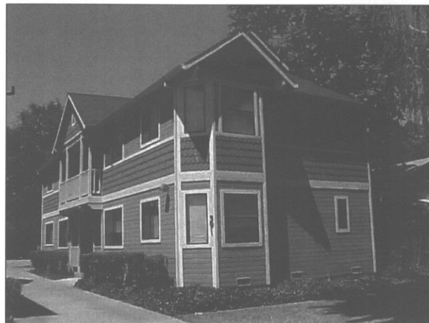
Windows and doors should be of a traditional size and should be placed in a similar solid-to-void relationship as historic buildings. (San Jose, CA)
