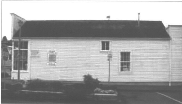
False fronts appear on surviving commercial type buildings. These conceal gable roofs.
