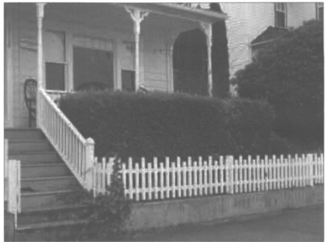
Fences and walls should be designed to allow views into a yard while at the same time successfully defining one's property line.
