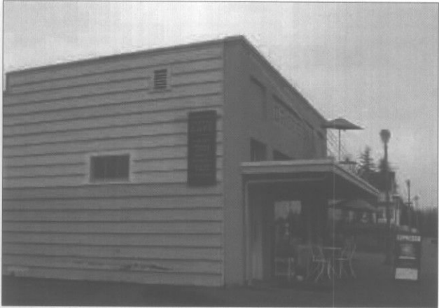
The Grocery Store has a stepped parapet roof and wood clapboard siding.
