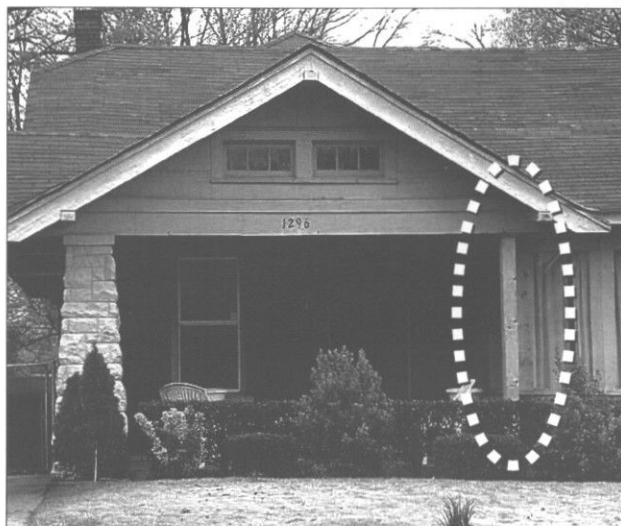
Preserve an original porch. Avoid using a porch support that would be substantially smaller than other supports on the porch or than seen historically. (Memphis, TN)
