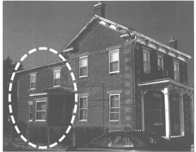
Appropriate: Preserve an older addition that has achieved historic significance in its own right. (Sainte Genevieve, MO)
