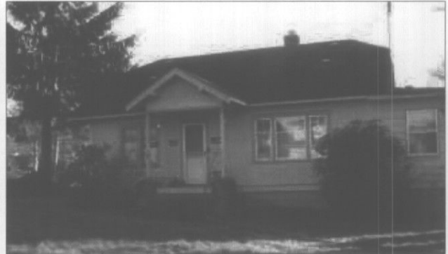
Most entrances are raised above the site grade and are defined by steps.
