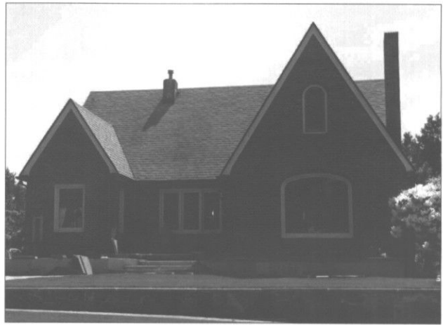
Typical Tudor Revival characteristics include a steeply pitched roof and the use of brick.
