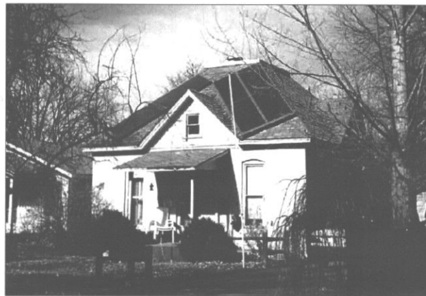
The addition of features such as skylights or solar panels should not be installed in a manner such that they will interrupt the plane of the historic roof. (Ft. Collins, CO)
