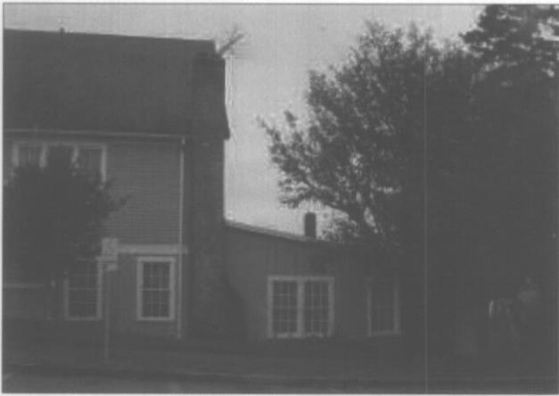
The rear addition to the former Oberlin Congregational Church (c. 1903) is simple in design and can be recognized as both a product of its own time and simple in character. (Steilacoom, WA)
