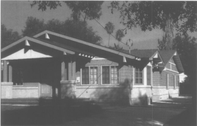
Subdividing a larger building mass into smaller “modules” that are similar in size to buildings seen traditionally is encouraged. This new house is divided into modules, which is appropriate. (Pasadena, CA)
