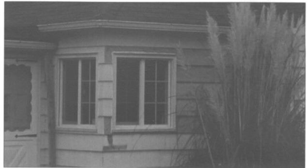
Retain and preserve original wall and siding materials.
