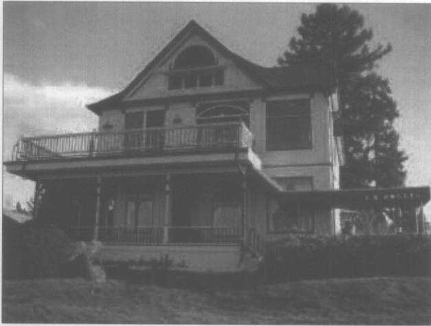
The E. R. Rogers House is a multi gable Queen Anne with shiplap siding and shingle wrap around the upper window openings. (c. 1893)
