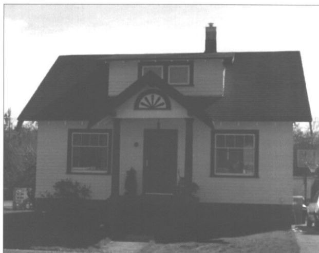
The two Steilacoom homes in the images above exhibit elements of the Craftsman style including exposed rafters, porches, and clapboard siding.
