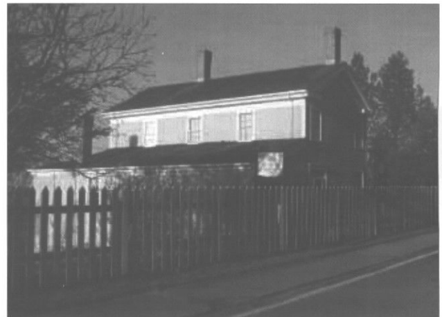
The Nathaniel Orr Home is on the National Register and has a gable roof and cornice returns with a single story shed addition built to the side. (c. 1857)
