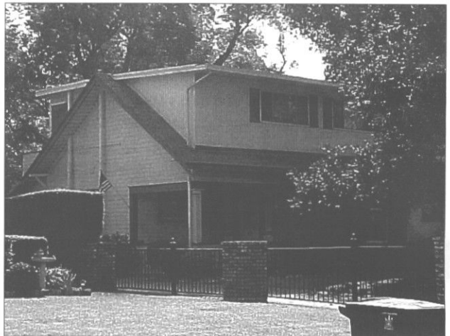
Inappropriate: A new dormer should remain subordinate to the historic roof in size and character. The dormers on the front and rear of this structure are too large and are inappropriate. (Memphis, TN)
