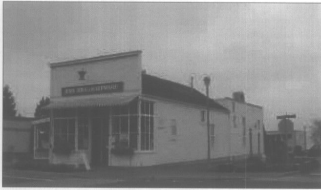
Bair's Store was built in 1895 with a false front. It has a stepped parapet roof and wood clapboard siding.
