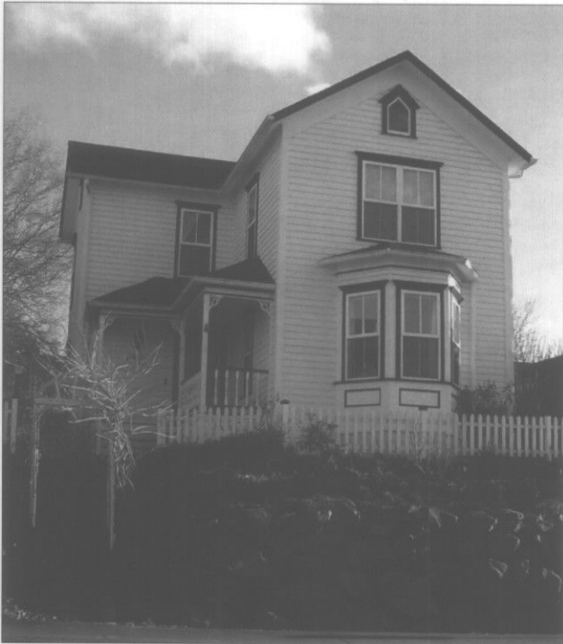
The Rigney House is a two-story Queen Anne with 2/2 single and paired double hung sash windows and a bay window on the ground floor. (c. 1880)
