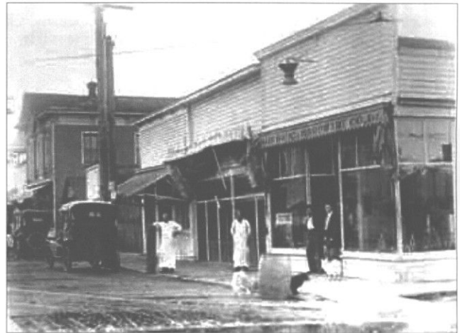
The town's early commercial buildings were basic woodframe structures with traditional false front architectural detailing.
