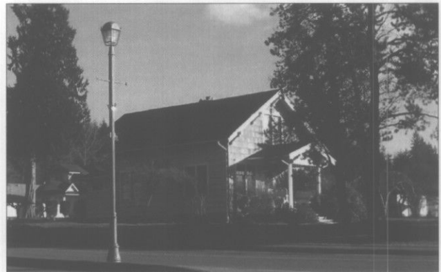
The primary entrance is typically defined by a porch or stoop.
