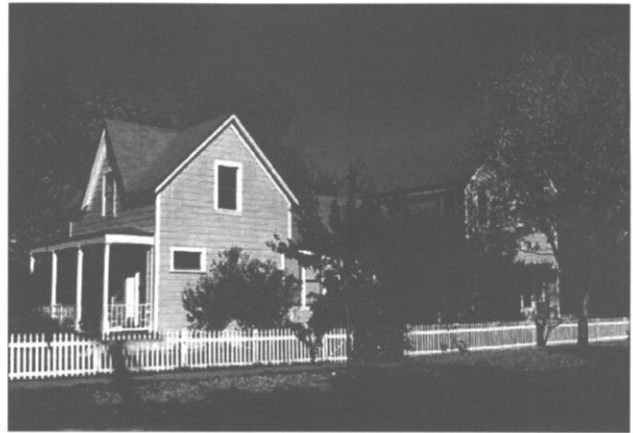
Appropriate: Design an addition to be compatible in size and scale to the main structure. This addition appears to be in scale with the original structure because it is separated with a smaller connecting structure. (Napa, CA)
