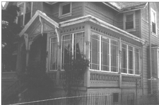
Appropriate: Where a porch must be enclosed, use transparent materials and place them behind the balusters and balustrade to preserve the visual character of the porch. (San Jose, CA)
