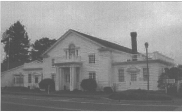
The Steilacoom Town Hall, built in 1930, exhibits Greek Revival elements including the portico over the front door supported by columns and the Palladian window above the entry.
