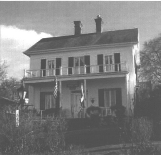
The Phillip Keach Home, also known as Rolling Hill, was built in 1858. It exhibits Greek Revival elements such as a full width entry porch supported by columns and tall first floor windows, as well as a transom and side lights surrounding the front door.
