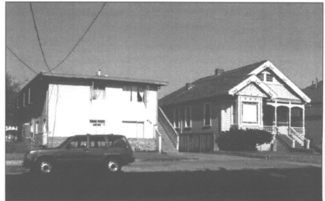
Pitched gable and hip roofs are encouraged where they exist on surrounding historic houses. The structure to the left in the photo is inappropriate.
