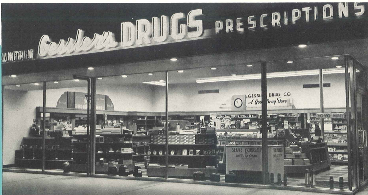
Location: Wichita, Kansas. Architects: Forsblom & Parks, Wichita. Products Used: Pittsburgh Polished Plate Glass; Carrara Structural Glass; Pittco Store Front Metal; Herculite Tempered Plate Glass Doors.
