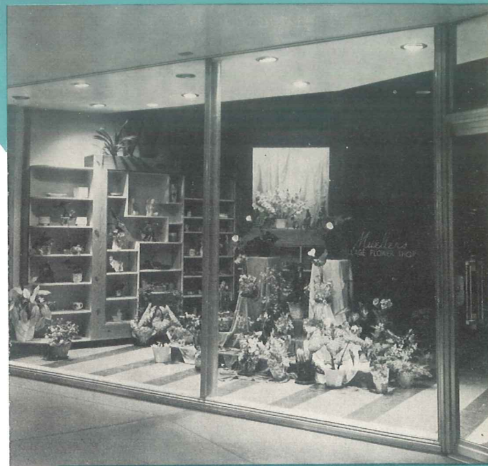
Location: Wichita, Kansas. Architects: Forsblom & Parks, Wichita. Products Used: Pittsburgh Polished Plate Glass; Carrara Structural Glass; Pittco De Luxe and Pittco Premier Store Front Metal; Herculite Tempered Plate Glass Door.
