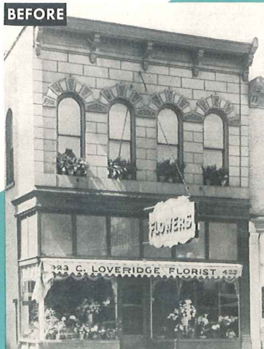
Location: Peoria, Ill. Architect: Cletis R. Foley, Peoria. Products Used: Pittsburgh Polished Plate Glass; Pittco De Luxe Store Front Metal; Herculite Tempered Plate Glass Door.
