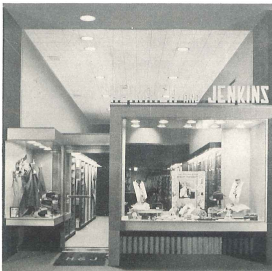
Location: Cumberland, Md. Architect: S. Russ Minter, Cumberland. Products Used: Carrara Structural Glass; Pittsburgh Polished Plate Glass; Herculite Tempered Plate Glass Door; Herculite Door Frame Assembly; Pittco De Luxe Store Front Metal.
