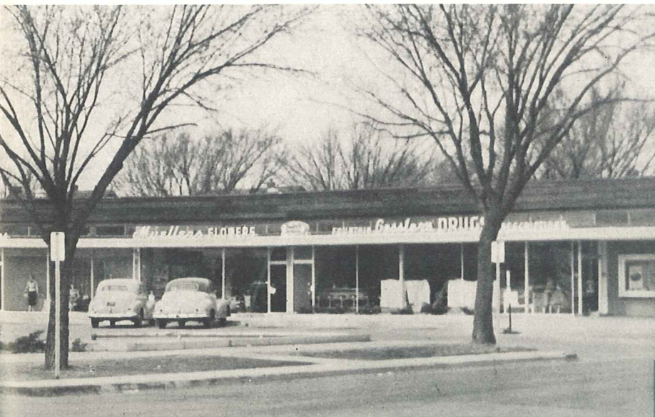
Location: Wichita, Kansas. Architects: Forsblom & Parks, Wichita.
