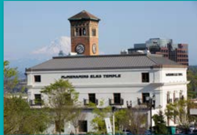
McMenamins ELKS Temple in Tacoma was restored with the assistance of the Federal Rehabilitation Tax Credit program. Photo Kathleen Nyberg
