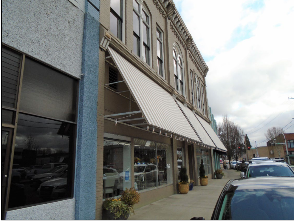
Photograph 3. Primary façade of the Newell Hunt Building, facing east (Stantec 2023).
