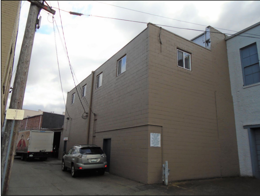
Photograph 5. Rear façade of the Newell Hunt Building, facing southeast (Stantec 2023).
