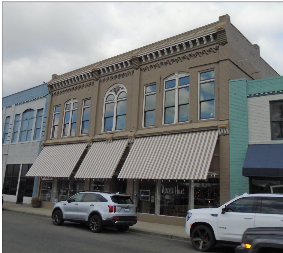
Photograph 2. Primary façade of the Newell Hunt Building, facing northwest (Stantec 2023).
