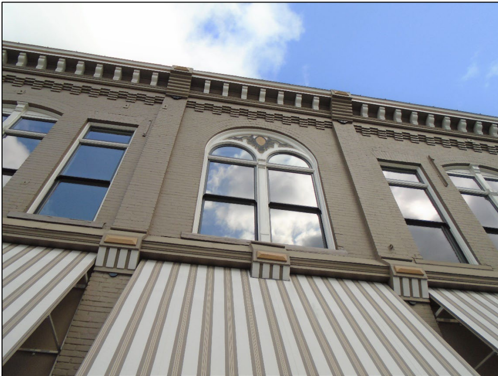
Photograph 4. Decorative Italian Renaissance Revival elements on the primary façade of the Newell Hunt Building (Stantec 2023).
