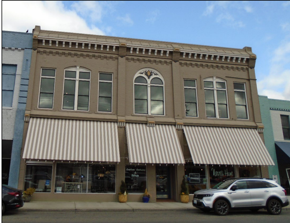
Photograph 1. South-facing primary façade of the Newell Hunt Building, facing north (Stantec 2023).
