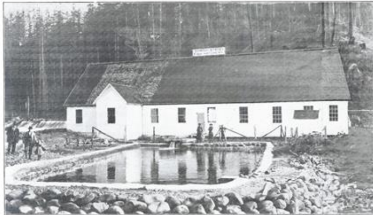
Samish salmon hatchery, showing new concrete rearing ponds.
