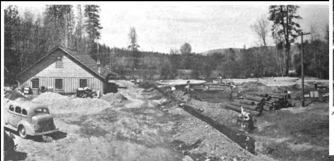
Panorama view of new Spokane hatchery construction. (Left) Hatchery building. Seventeen standard 40-foot concrete rearing pools are now in operation here.
