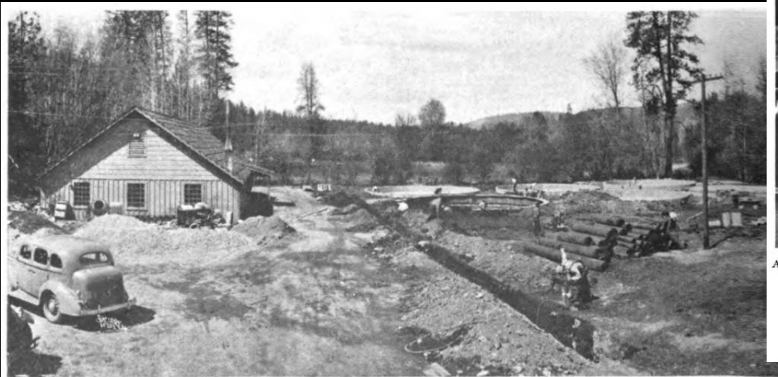
Panorama view of new Spokane hatchery construction. (Left) Hatchery building. Seventeen standard 40-foot concrete rearing pools are now in operation here.
