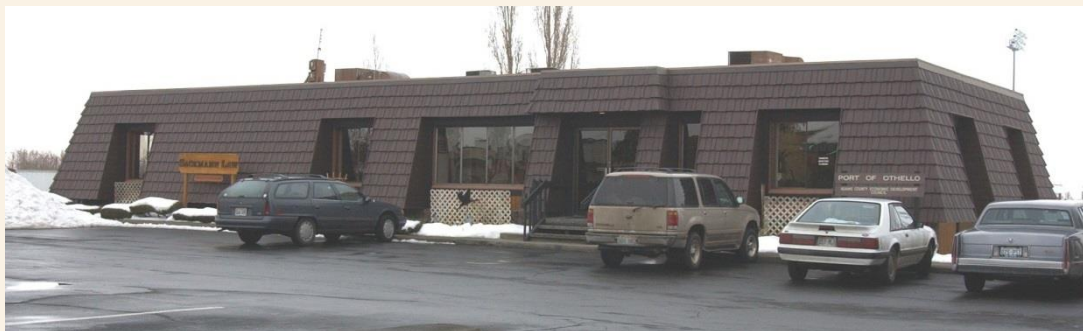
BUILDING | OTHELLO, C.1972
