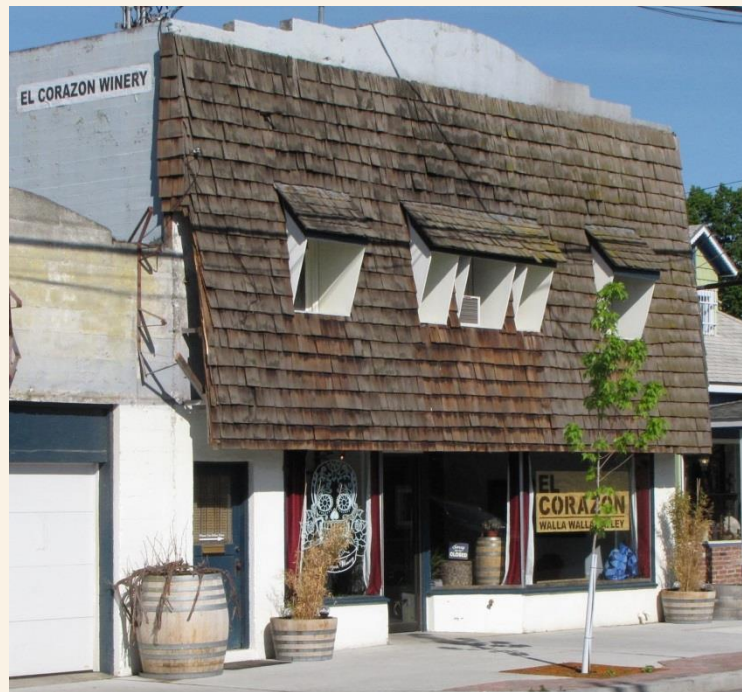
BUILDING | WALLA WALLA, C.1978
