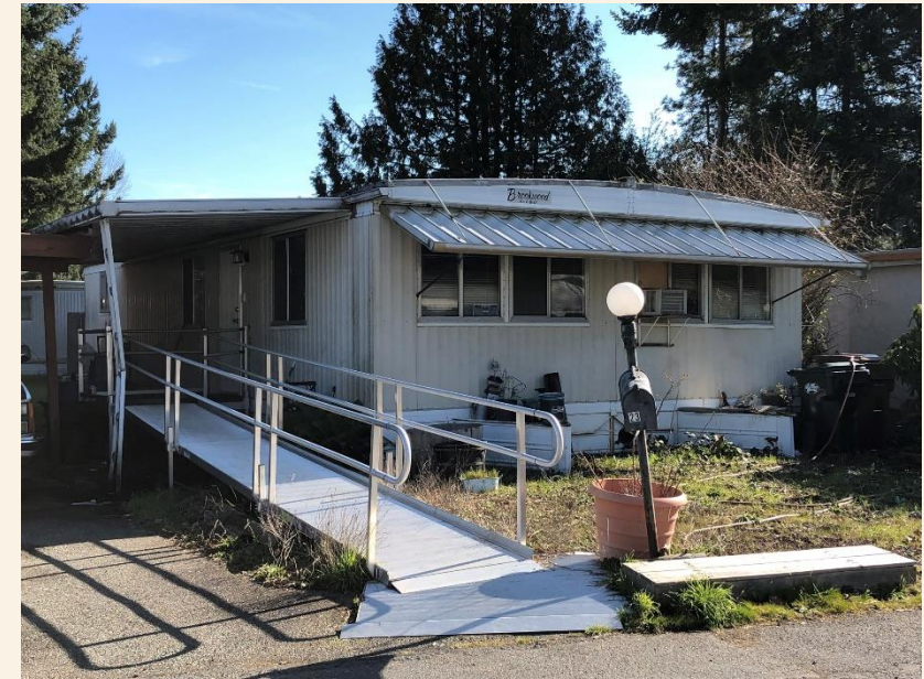
WINDSOR COURT MOBILE HOME ESTATES | TACOMA
