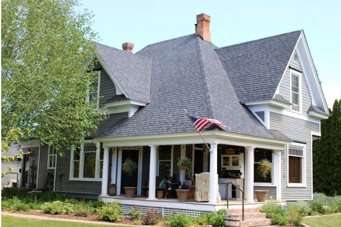
1. Looking northeast at Kincaid-Daling House west and front elevations.
