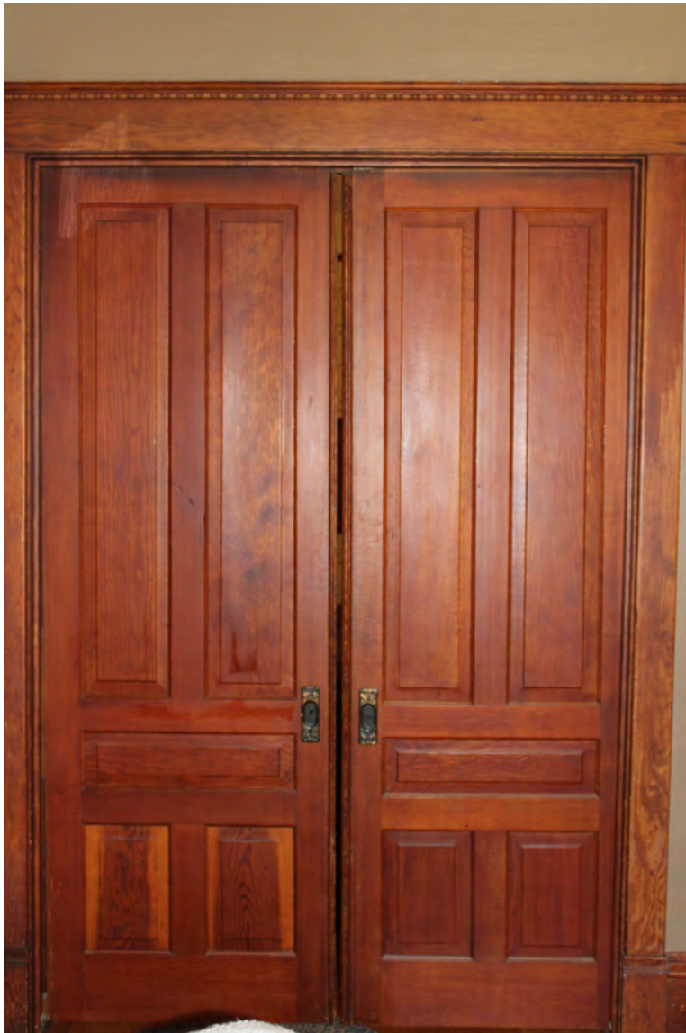
13. Pocket doors in Kincaid-Daling House between original parlor and dining room.
