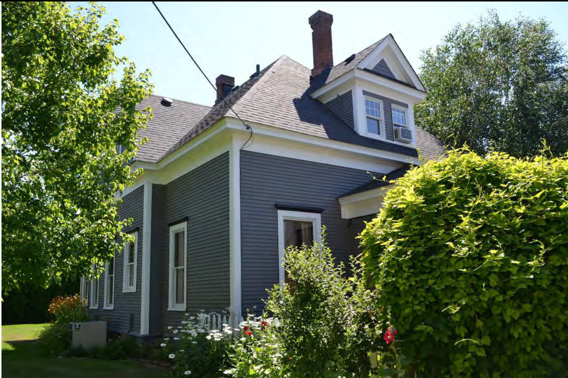
5. Looking south at east and rear elevations of Kincaid-Daling House. Photograph by Ann Sharley July 2021.
