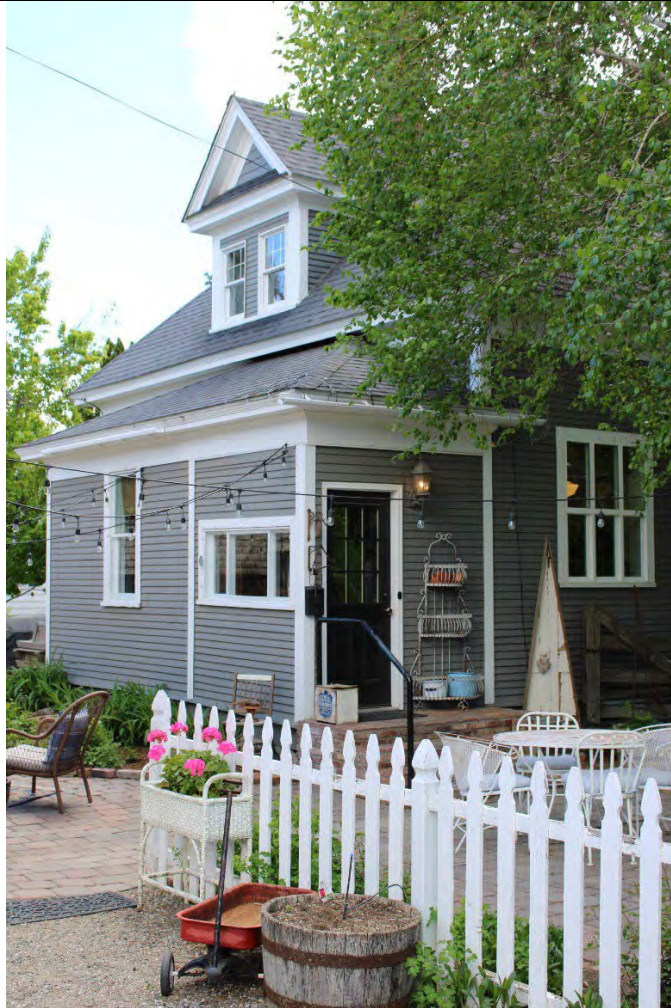
7. Looking southeast at rear elevation of Kincaid-Daling House.
