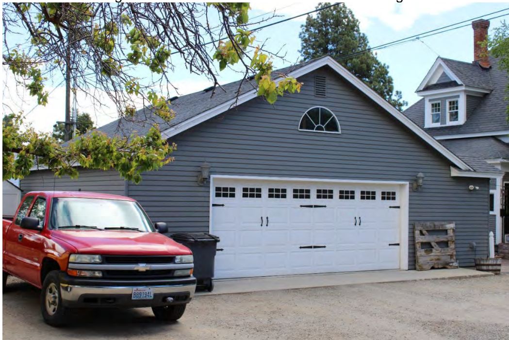
8. Looking southeast at the new garage's front elevation.
