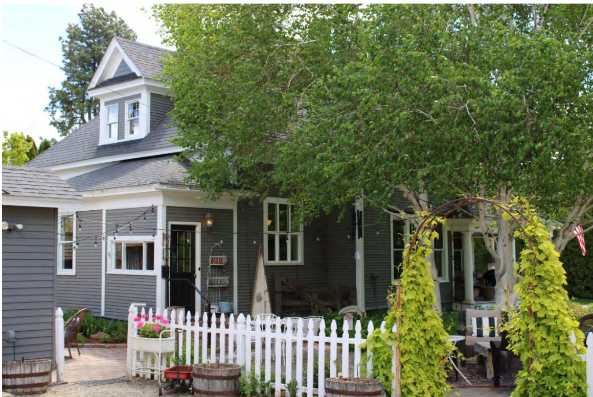
6. Looking southeast at rear and west elevations of Kincaid-Daling House.
