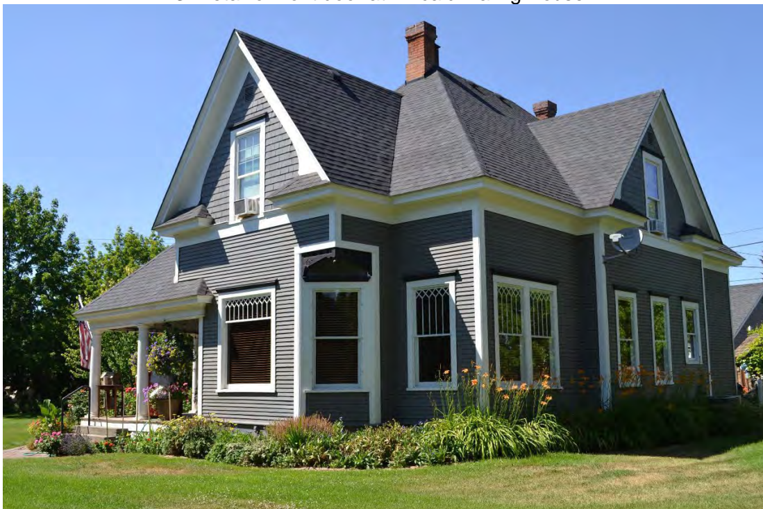
4. Looking northwest front and east elevations of Kincaid-Daling House. Photograph by Ann Sharley July 2021.
