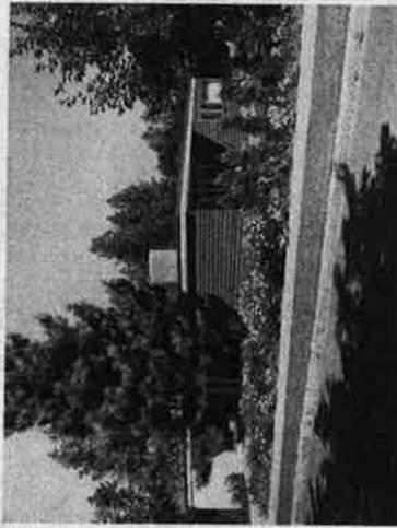
This Five Star home is easily built, easily maintained. It's only 9 feet from inexpensive concrete slab up to simple built-up roof (flat over dead-level beams). Many folks would stain flat-floor and paint or stain this 8 feet of lap siding. Windows are simple to clean, too. Perfectly flat awn; flush roof furthers simplicity, economy of design.
