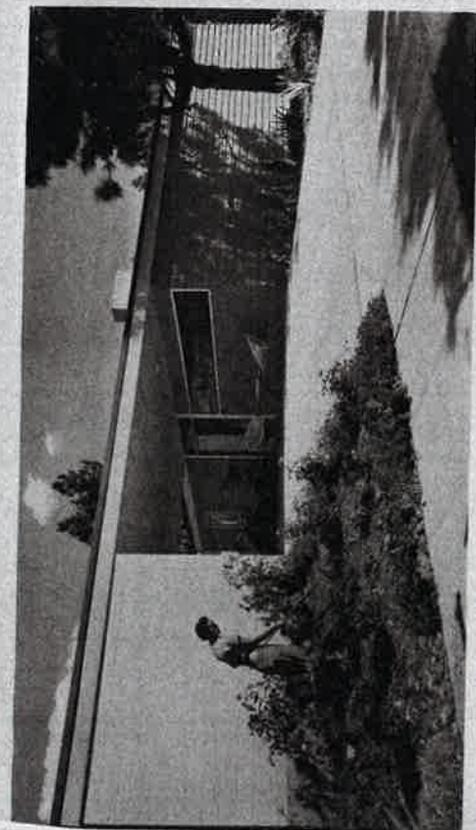
Precise, rectangular house turns blank wall toward street (or whatever view you care to minimize). Carport and storage room shield house from closely bordering neighbors. Built on a slab, storage room takes place of basement. Carport doubles as shelter for front door, also shades front terrace. Strip window under carport gives light, ventilation to living area, yet allows privacy.
