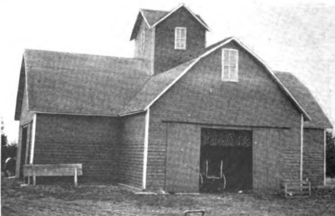
**Fig. 3.** Plan and photograph of a cross-shaped farm elevator having two driveways intersecting at right angles. The driveways occupy an excessive amount of space in proportion to storage capacity
