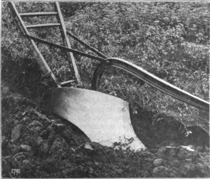
Fig. 10. Plow pulled back, showing that no earth stuck to the moldboard
