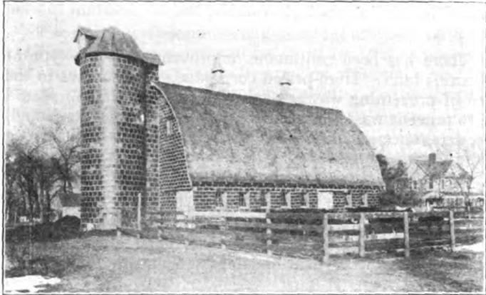
Gothic arch roof construction on a clay block barn
