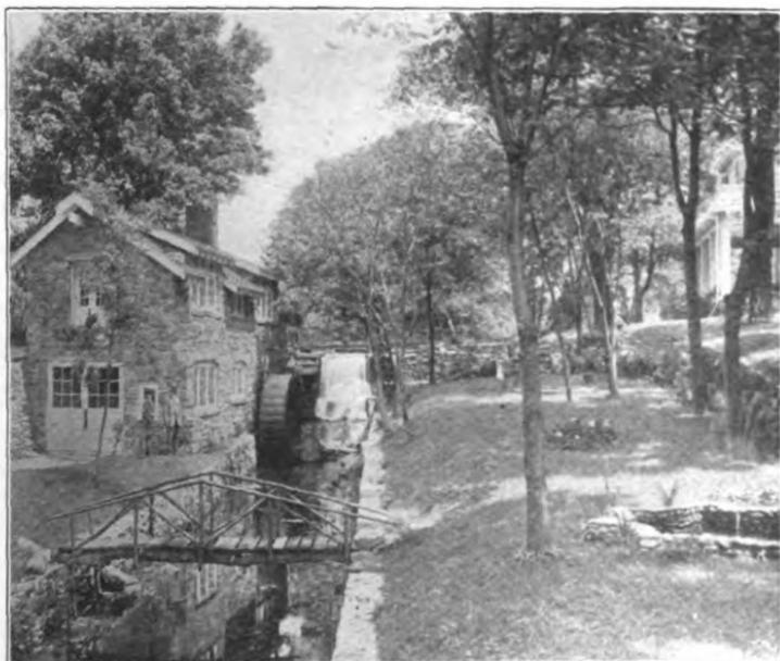
Fig. 7. Wheel installed at dam, saving cost of raceway and pipe
