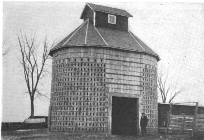
Fig. 5. A concrete stave farm elevator with semi-circular cribs and bins for small grain over driveway
