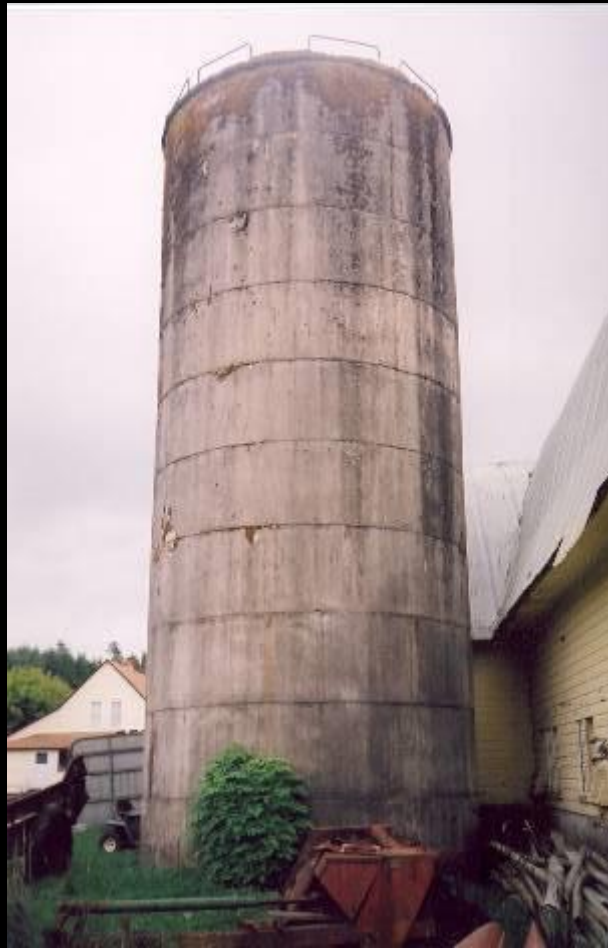
Poured Concrete Silo
