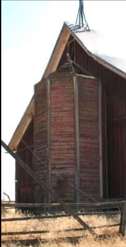
Wooden Octagonal Silo
