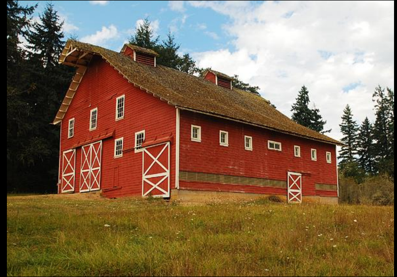
Finley National Wildlife Refuge, Benton County, OR
