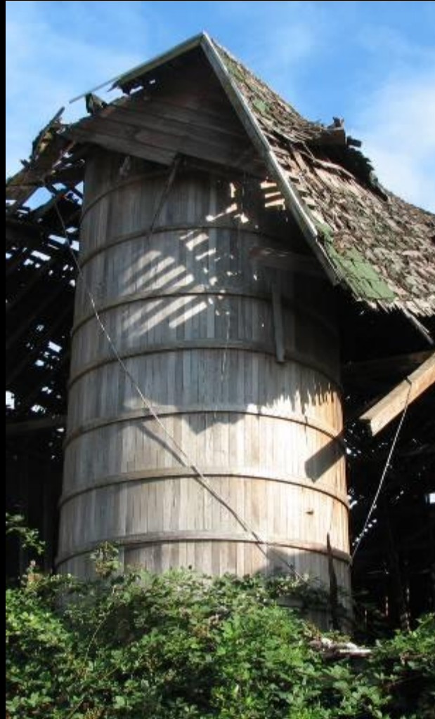
Vertical Wood Stave Silo
