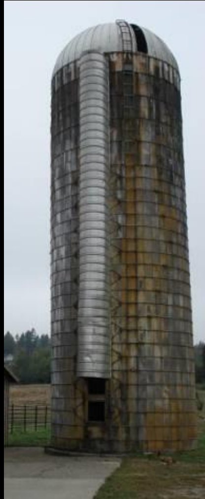
Concrete Stave Silo Pierce Co. – c.1920
