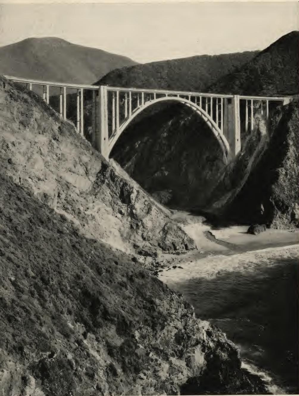
*Bixby Creek Bridge on Carmel-San Simeon Highway, Calif., has 320-foot span and 240-foot height over stream bed. Designed by California State Highway Commission under direction of C. H. Purcell, now State Highway Engineer. A good example illustrating a beautiful arch line, large piers defining the ends of arch span, piers as well as spandrel columns showing proper inflection by means of tapered and offset lines.*
