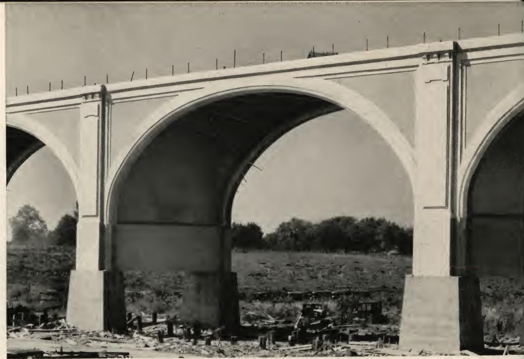
*Vachel Lindsay Memorial Bridge at Springfield, Ill., crosses an area that was later to be inundated. Semi-elliptical soffit curves are accentuated by a design cast in plaster waste molds. Design by Burns and McDonnell, Kansas City, Mo.*
