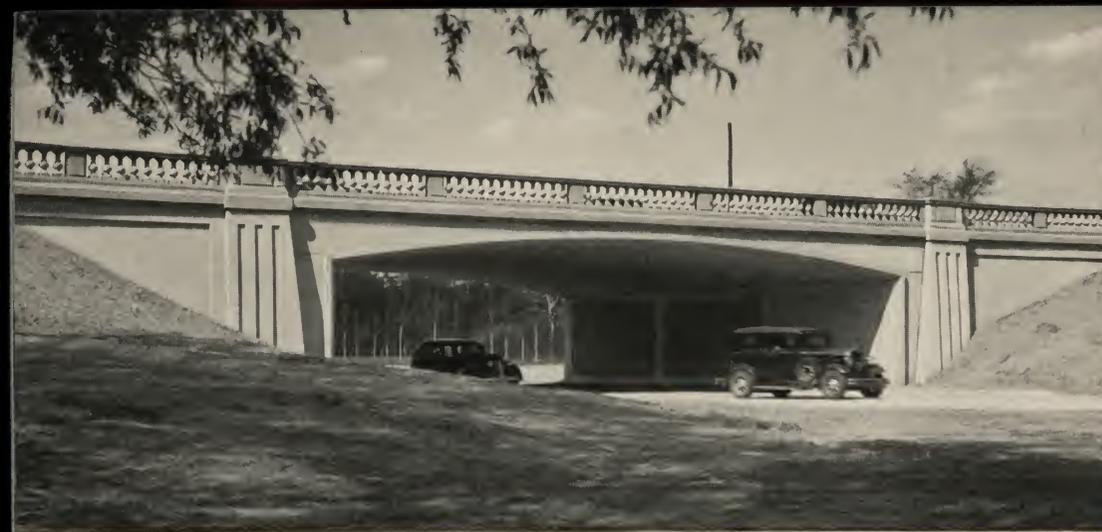
*Rigid frame structure separates Plymouth Road and Middle Rouge Parkway in Wayne County, Mich. Design by Wayne County Road Commission, H. A. Shuptrine, Bridge Engineer. The pilasters are designed with a battered line on the side toward the span in order to mark the outline of the rigid frame, which is made the focus of interest.*
