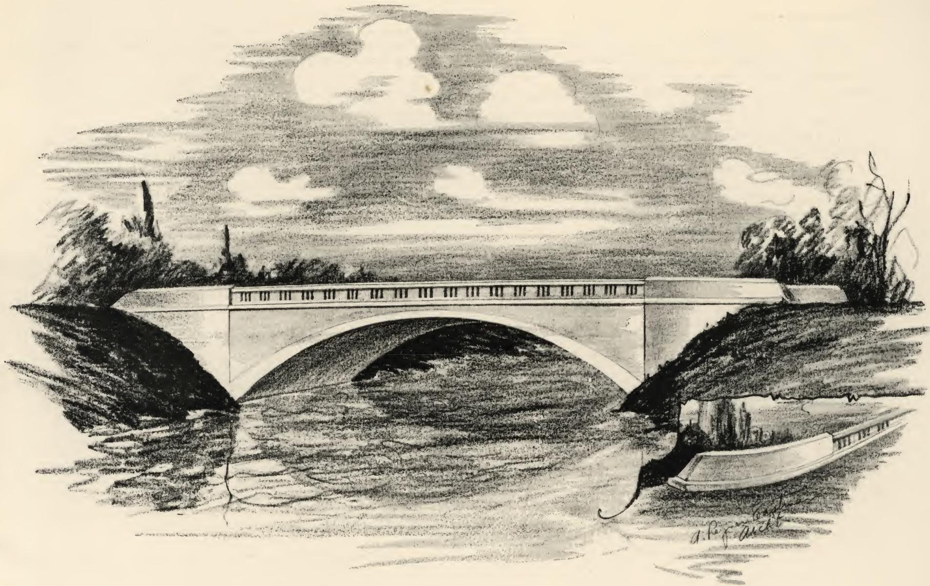
*The spandrel-filled arch bridge, drawn by A. Reyner Eastman, has a segmental soffit curve of decisive quality. The water table line expresses unity in the structure itself as well as unity with the highway grade line as a whole. Slightly increased height of parapet on wing walls with solid and flared construction imparts inflection, strength and stability to the appearance of abutments.*
