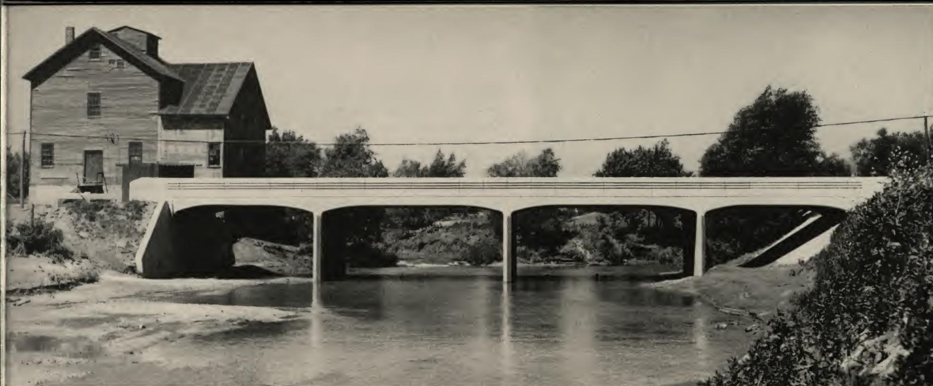
*Multiple-span rigid frame bridge over Leaf River in Ogle County, Ill., built in 1937 and designed by Mogens Ipsen, Rockford, Ill. Horizontality is strongly emphasized by the parapet design which gives the structure a distinctive sense of unity and diverts attention from the dissymmetry of the abutments.*
