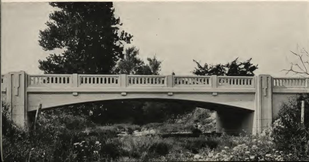
*Rigid frame bridge, designed by Carl Kuch, carries Findlay-Delphos Road over Cranberry Creek in Putnam County, Ohio. The segmental soffit curve is the center of interest and makes the structure appear higher than if the soffit had been made straight. The vertical design of pilasters and posts serves to accentuate height, an important consideration in a structure with long span but shallow headroom.*
