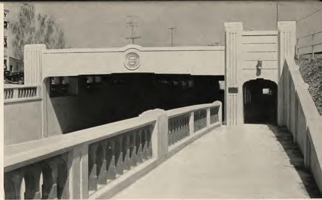
*Close-up of grade separation structure in Salem, Ore., illustrates that beauty may be expressed by simple architectural design. Note offsets in soffit line over pedestrian tunnel, the same motif being used in the roadway span. The lack of symmetry does not disturb the effect of the design.*
