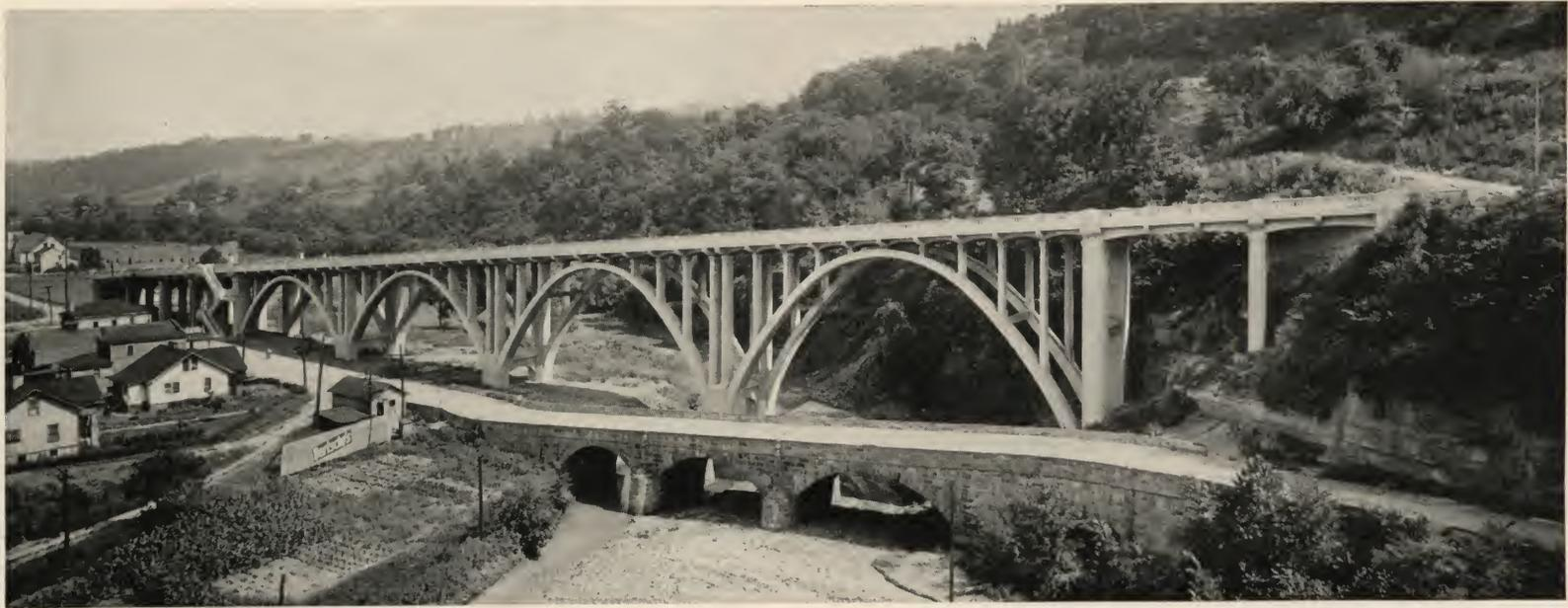
*Blaine Viaduct at St. Clairsville, Ohio, is also referred to as "Arches of Memory." Built in 1933 and designed by Ohio State Department of Highways and Public Works, J. R. Burkey, Chief Engineer of Bridges. The roadway grade dictated a design with arch spans varying from 103 to 146 feet, and the gradual increase in size of the arches lends interests to this unsymmetrical layout.*
