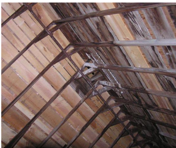
Exposed Replacement Skip Sheathing
