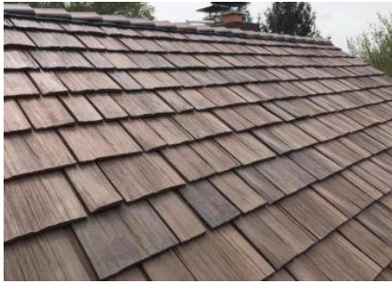
Not Allowed Treatment: Simulated Wood Shakes
