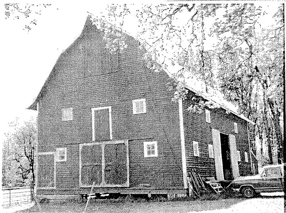
Figure 52. Gambrel-roofed barn with stud wall construction and timber purlin posts. The Kelly Barn built in ca. 1910.
