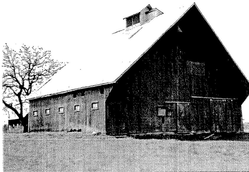
Figure 82. Hay Hoods. Ridge extended, peaked hay hoods (top and bottom). This hay hood form is generally found on gambrel roofed barns.
