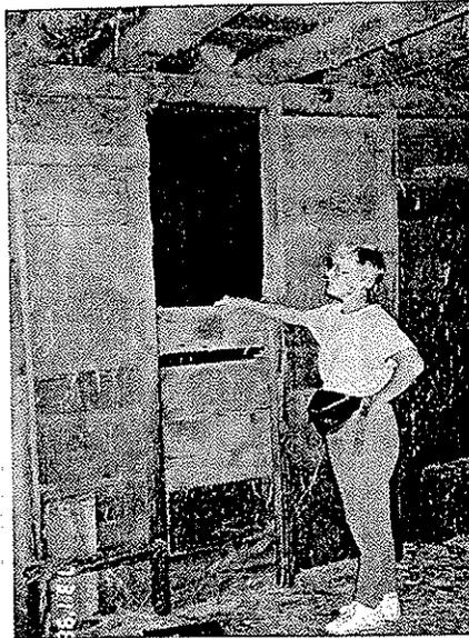
Figure 32. Grain bin opening with boards in slatted jambs.
