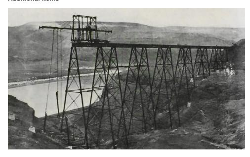
Description of Photograph: Typical method of erecting a bridge using a traveler, SP&S Box Canyon Viaduct.
