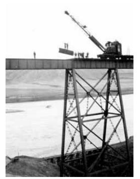
Description of Photograph: Replacing railroad ties on the SP&S Box Canyon Viaduct.
