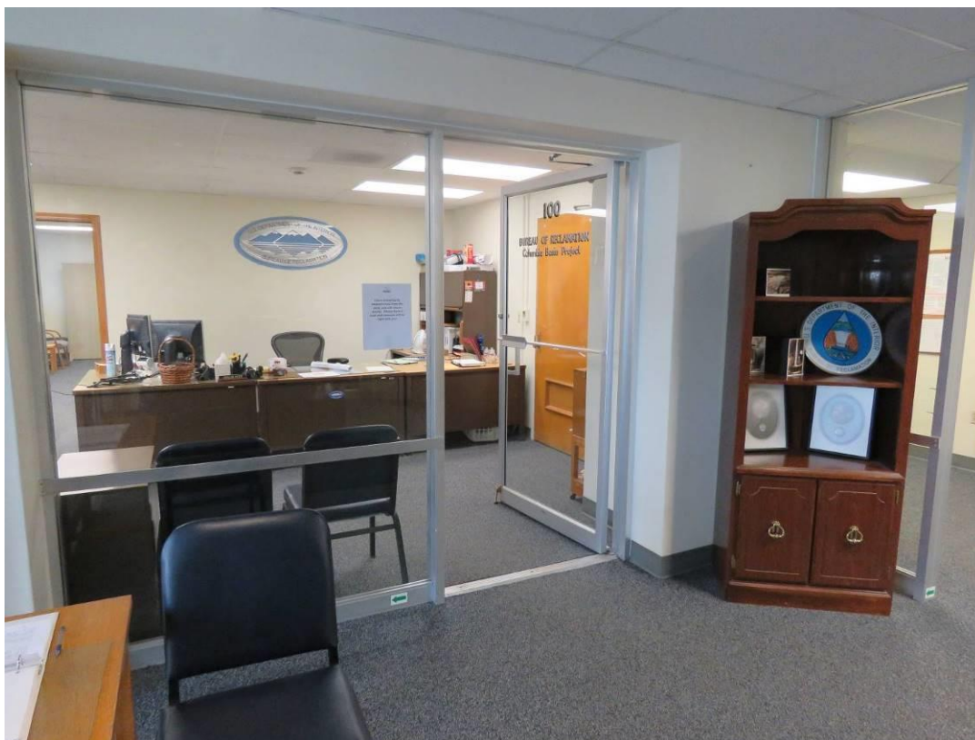
Photo No. 12 – Columbia Basin Project Irrigation Division Headquarters Office – View in First floor lobby looking north at 1960 remodel of glass and steel where a wall had been.
