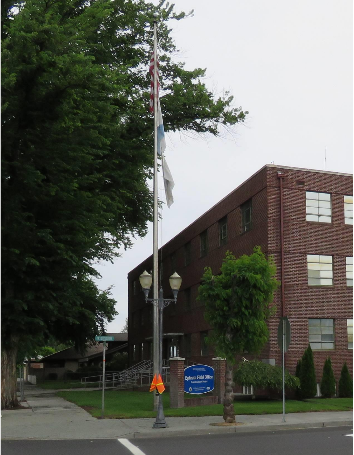
Photo No. 10 – Columbia Basin Project Irrigation Division Headquarters Office – View looking north at flagpole and modern sign for the building.
