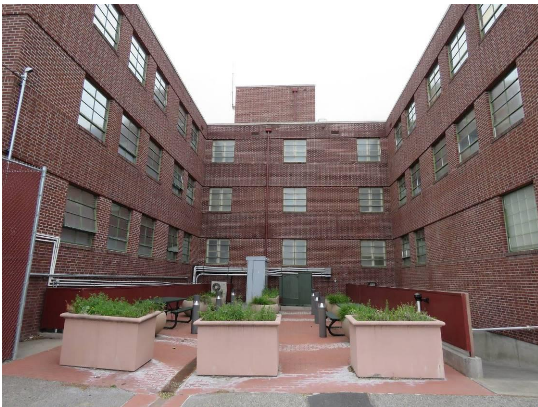
Photo No. 7 – Columbia Basin Project Irrigation Division Headquarters Office – Detail of the courtyard space within the U of the building's rear elevation.
