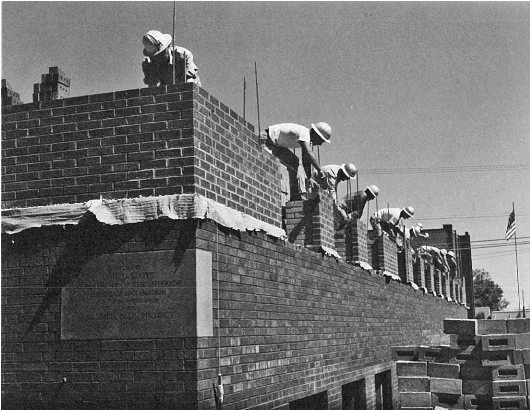
Brick masons working on the first floor of the Ephrata Office Building. Approximately 950,000 bricks are required. Reclamation Photograph No. 4-4183, August 3, 1950.
