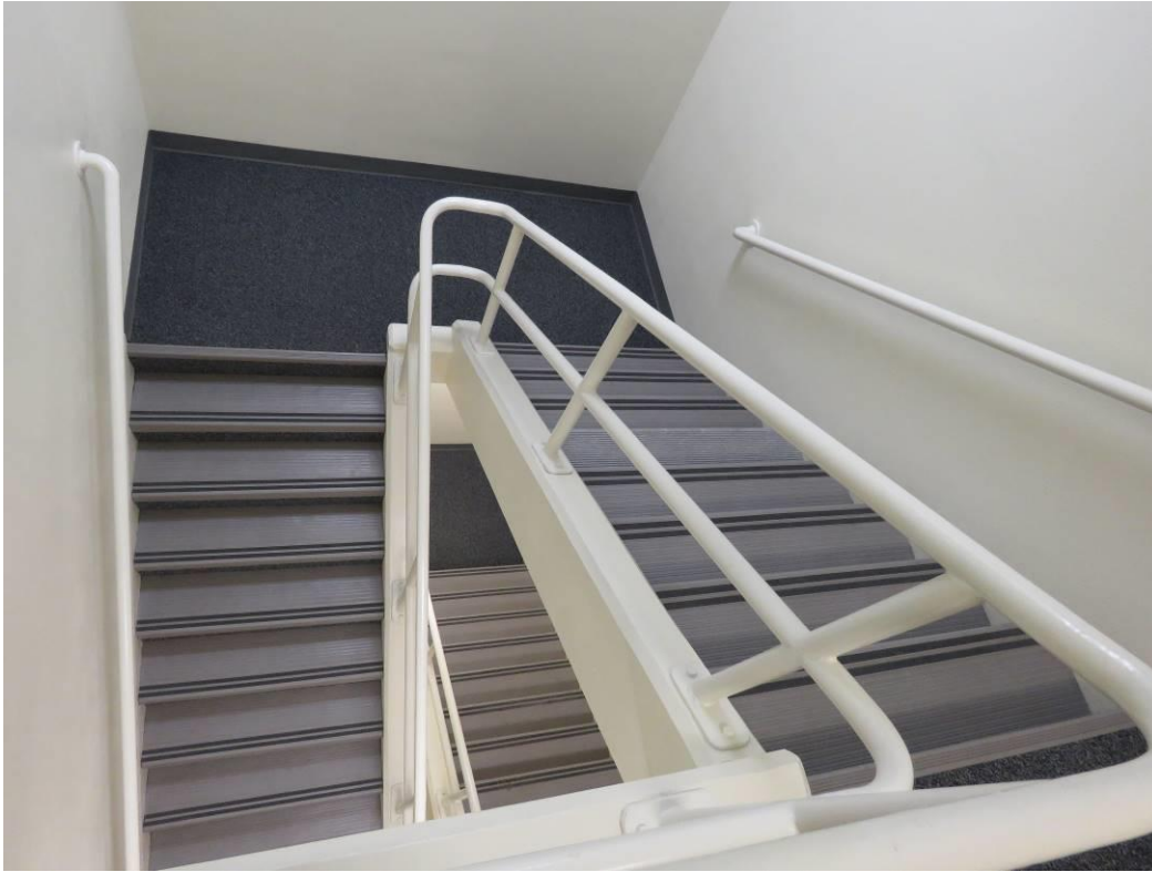
Photo No. 19 – Columbia Basin Project Irrigation Division Headquarters Office – South stairwell looking down from Third Floor.
