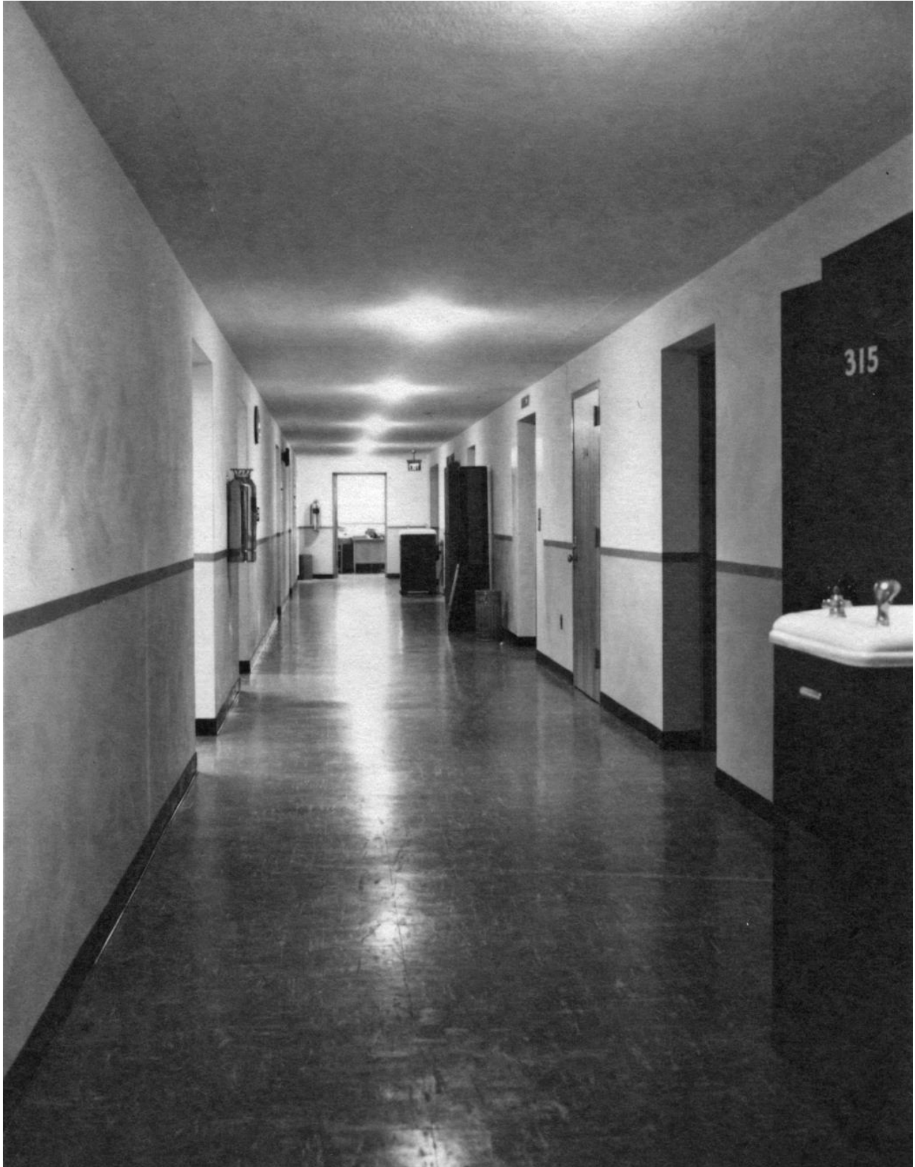
View of third floor corridor after completion of the building. Note the exposed wire on the ceiling which is a portion of the fire alarm system. Reclamation Photograph No. 31301, December 17, 1951.
