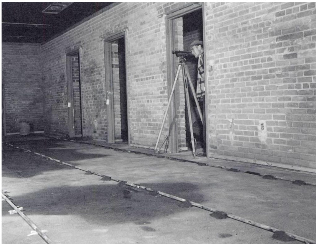
Instrument man leveling screeds in preparation for placing bonded concrete floor topping in the Ephrata Office Building. Reclamation Photograph No. 4-4680, January 3, 1951.
