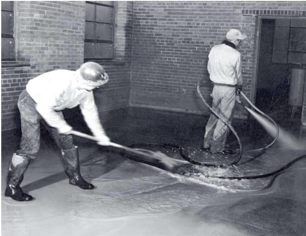
Clean-up crew cleaning structural concrete after sandblasting in preparation for placing bonded concrete floor topping in the Ephrata Office Building. Reclamation Photograph No. 4-4681, January 3, 1951.
