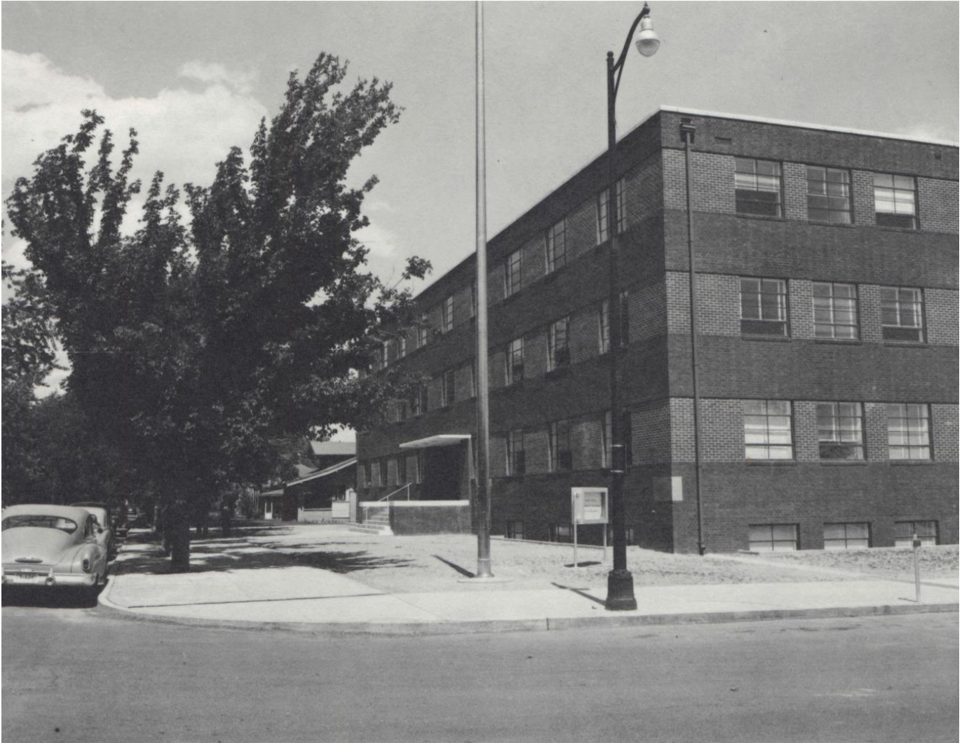
Completed building built to house the District Offices of the Irrigation Division. Reclamation Photograph No. 30274 July 10, 1951.
