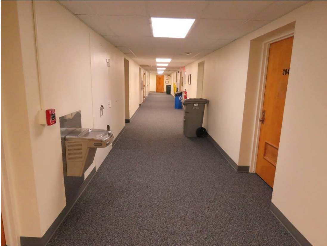
Photo No. 17 – Columbia Basin Project Irrigation Division Headquarters Office – Third Floor looking south.
