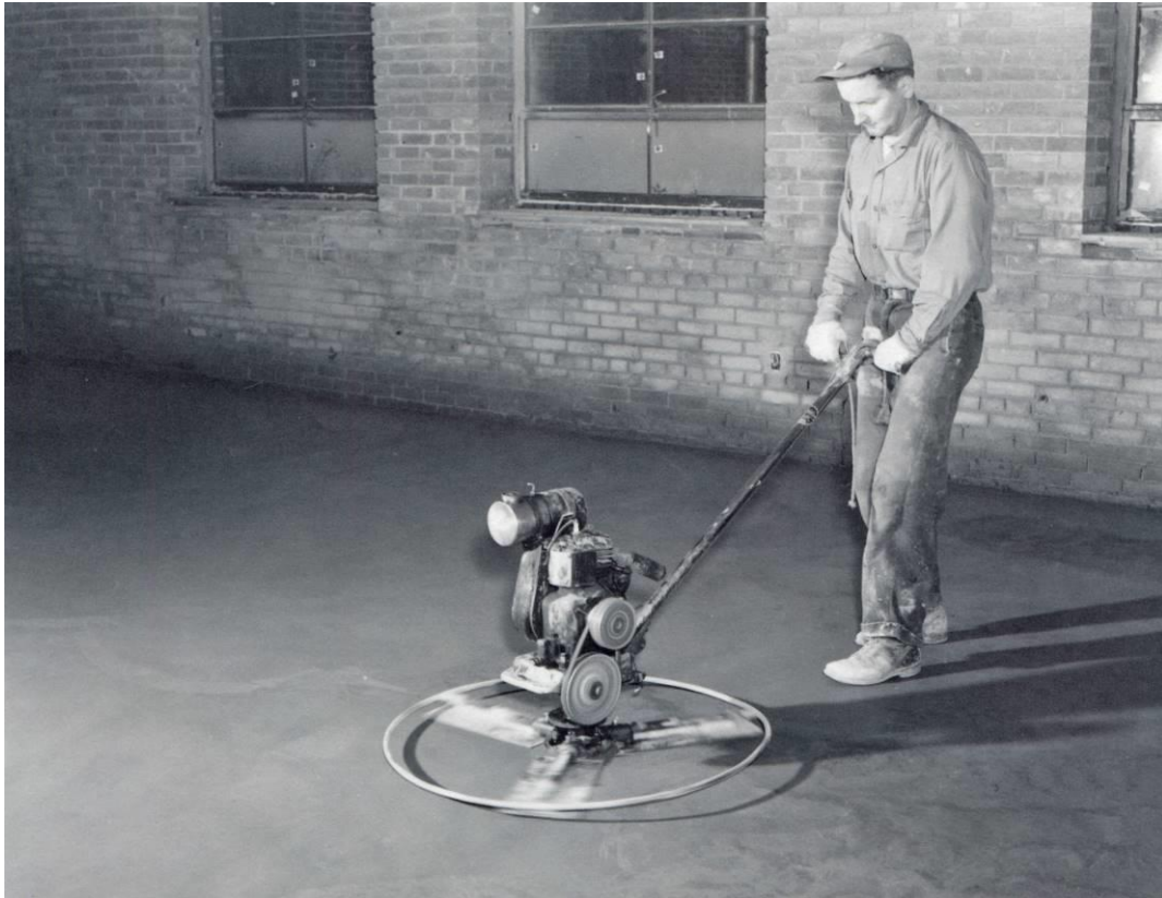
Concrete finisher operating power troweling machine on bonded concrete floor topping in the Ephrata Office Building. Reclamation Photograph No. 4-4679, January 3, 1951.
