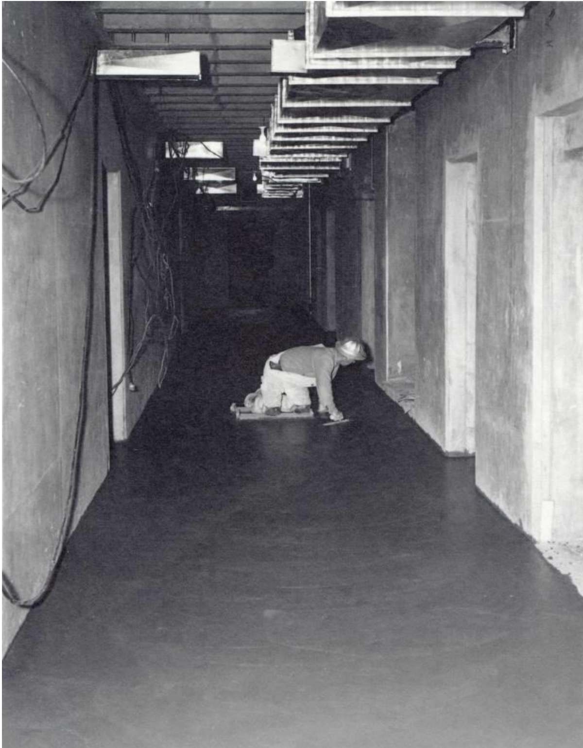
Concrete finisher finishing the floor in the basement corridor. Note ductwork at top of picture. Reclamation Photograph No. 4-4489, October 10, 1950.
