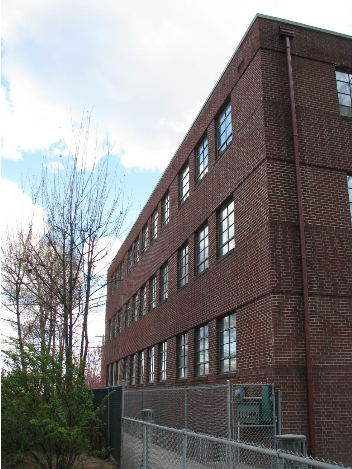
Photo No. 9 – Columbia Basin Project Irrigation Division Headquarters Office – Oblique view of North and a little of the Front Elevations. Photograph taken in 2012 by Kelsey J. Doncaster.
