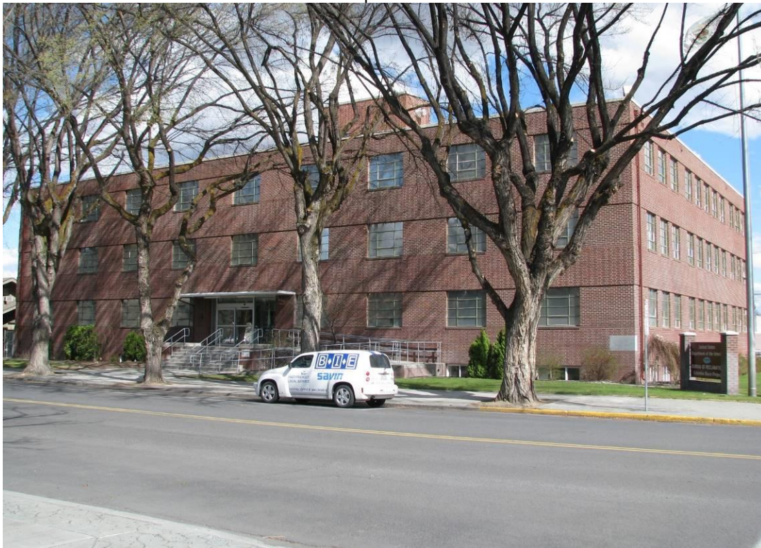
Columbia Basin Project Irrigation Division Headquarters Office – 2012 digital photograph by Kelsey J. Doncaster.
