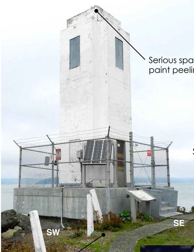
Serious spalling; paint peeling
