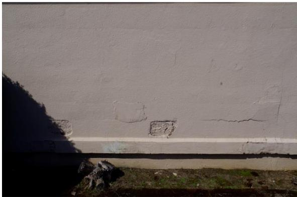
Exterior stucco cracks
