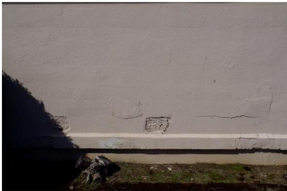
Exterior stucco cracks
