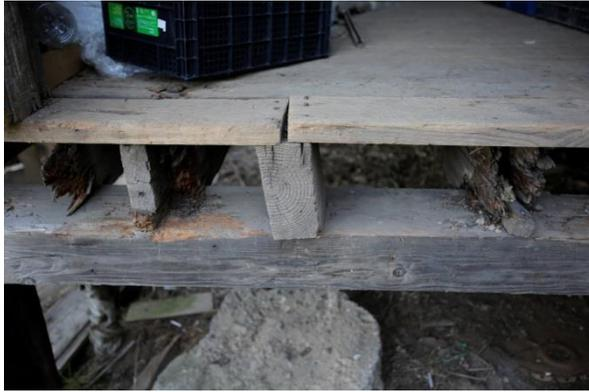
Rotting floor joists
