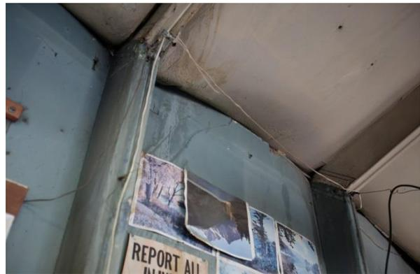
Warped and stained interior wall panels
