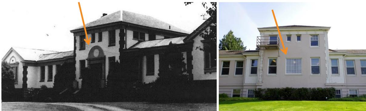
**Figure 43. Original front entrance facing 78th Street was infilled as an office space. Entrance details could be restored as an architectural feature.**
