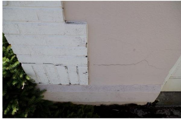
Structural cracking at the northeast corner
