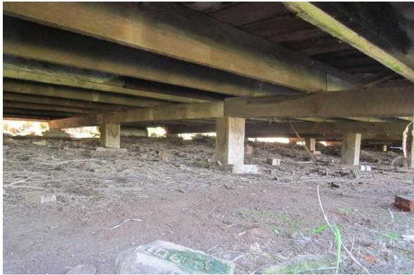
Bowing foundation beams
