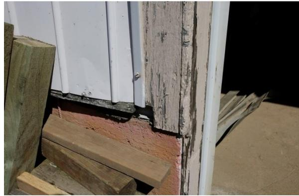
Deteriorated wood and peeling paint
