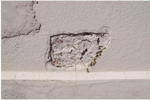
Exposed structural block on south elevation
