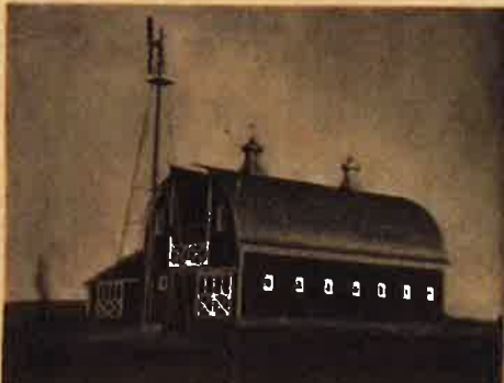
Circle roof barn of Mr. J. P. Walde, Warwick, North Dakota.
