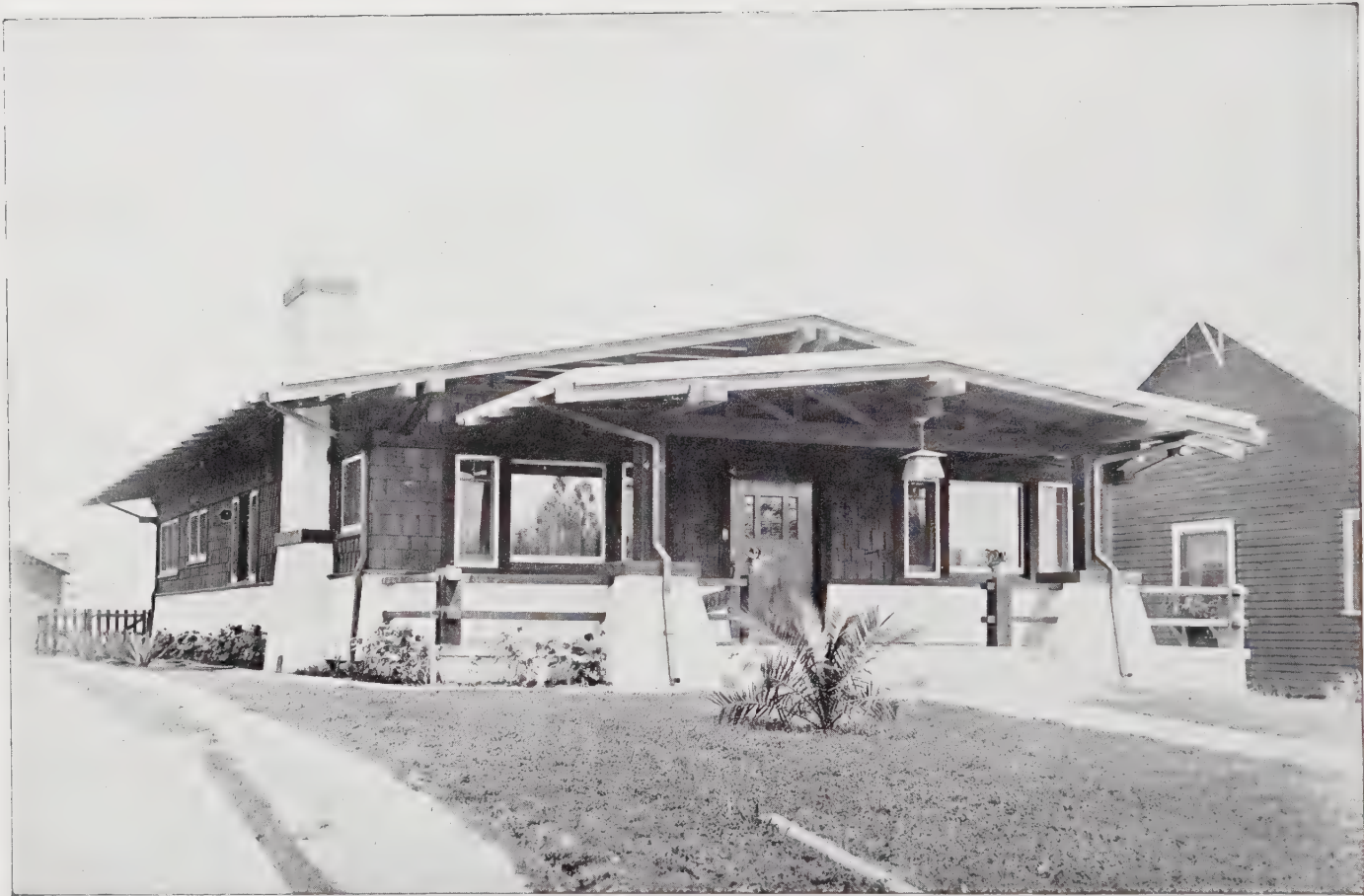
No. 456-A—THE CEMENT STUCCO BELOW THE WATERTABLE IS A PLEASING BIT OF DESIGN
