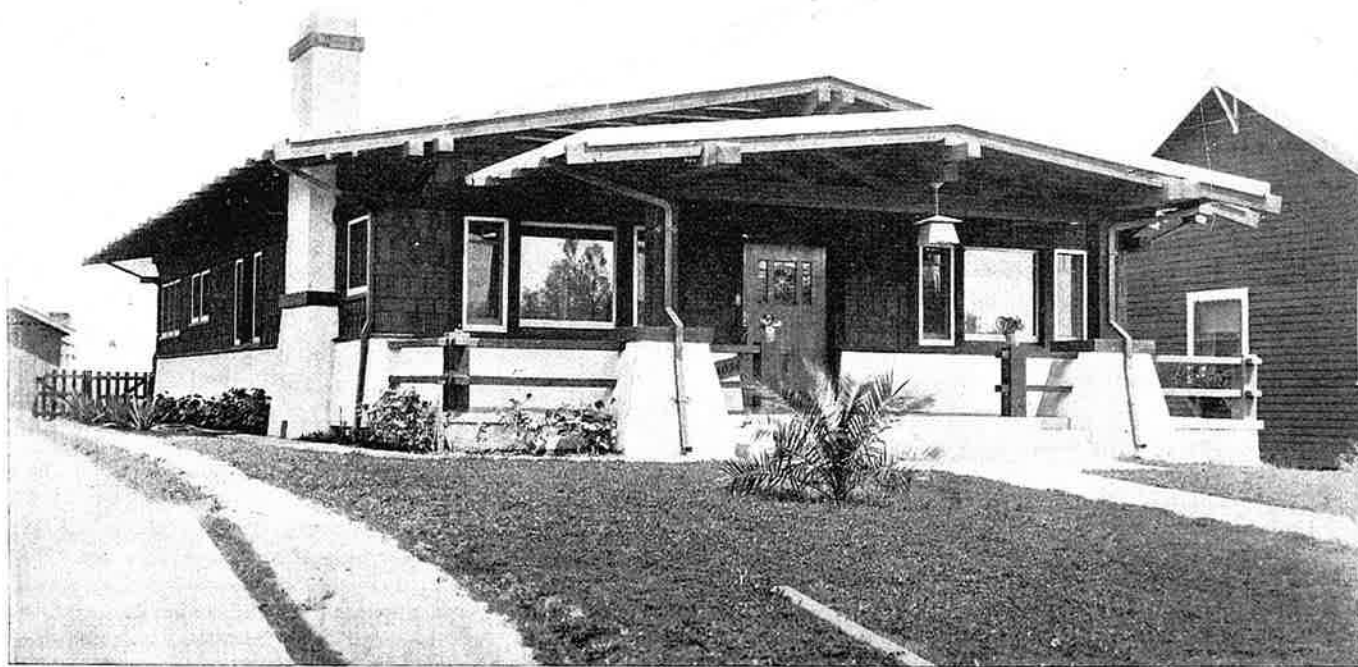
No. 456-A—THE CEMENT STUCCO BELOW THE WATERTABLE IS A PLEASING BIT OF DESIGN
