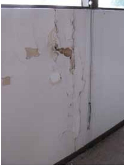
Detail of water damaged wall below northeast window, bedroom #2. Source: Artifacts Consulting, Inc. 2010
