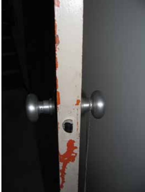
Basement bedroom door, showing added paint layer over original orange layer. Source: Artifacts Consulting, Inc. 2010
