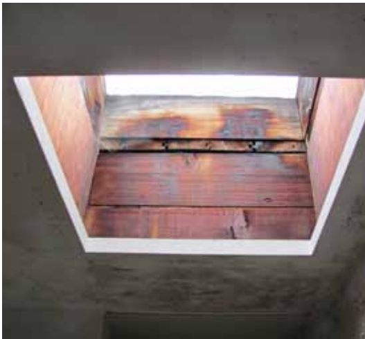
Detail of unfinished interior light well of skylight and mold on ceiling, bathroom #1. Source: Artifacts Consulting, Inc. 2010
