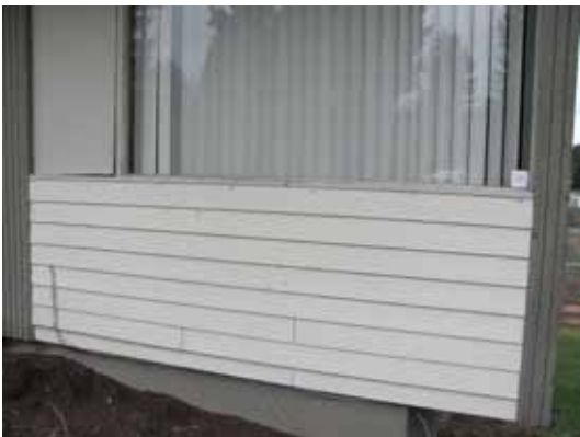
New horizontal veneer cladding beneath window of bedroom #3. Source: Artifacts Consulting, Inc. 2010
