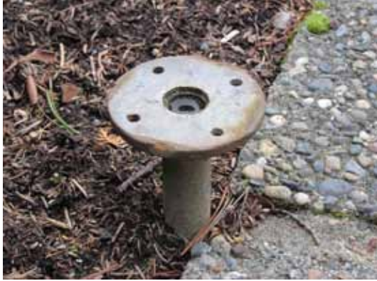
Detail of post support, indicating where a breeze-way wooden screen once stood. Source: Artifacts Consulting, Inc. 2010
