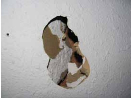
Detail of hole in wall of basement family room. Similar hole evident in bedroom #3. Source: Artifacts Consulting, Inc. 2010
