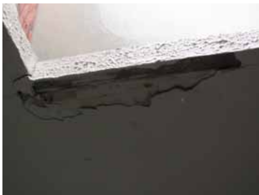
Detail of water damage at ceiling-light well junction in bathroom #2. Source: Artifacts Consulting, Inc. 2010
