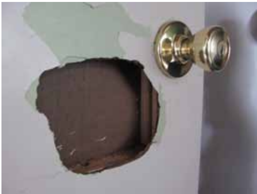
Detail of hole in door, bedroom #3. Source: Artifacts Consulting, Inc. 2010
