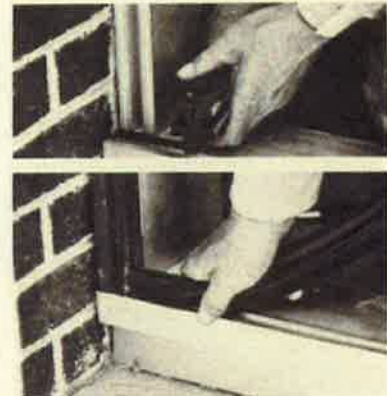
Gasket positioning
